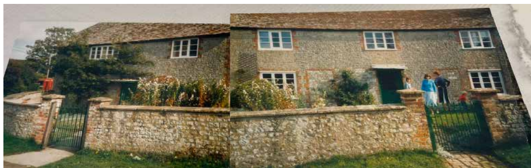
Fig 3 Photograph of Ashbys believed to have been taken around 1985, prior to approval W/87/01287/FUL
