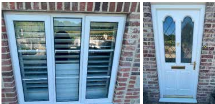
Fig 5 Existing PVCu window
