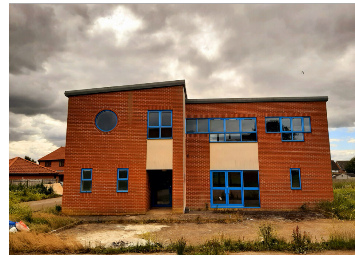
Existing Photographs- Block B
