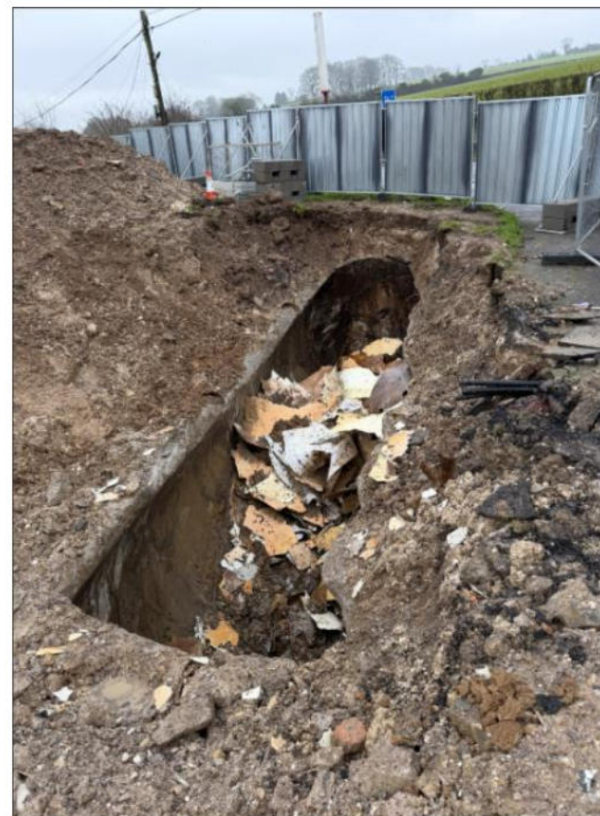
Breaking out of tanks in Trench 2
