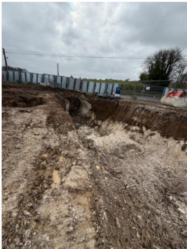
Deepened Trench 2 looking south
