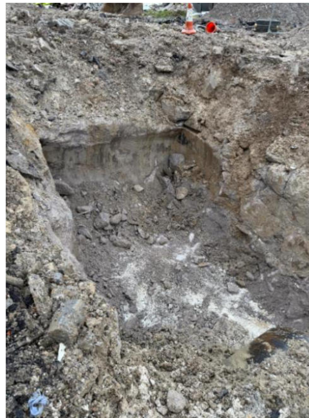
Breaking out of tanks in Trench 1
