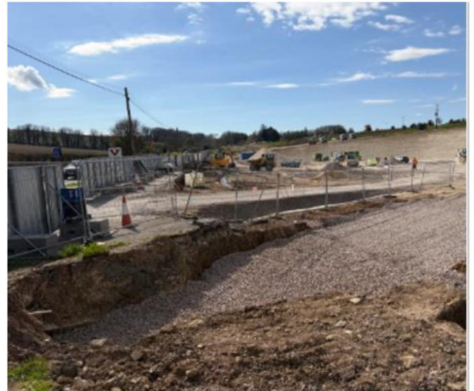
Backfilled Trenches looking north
