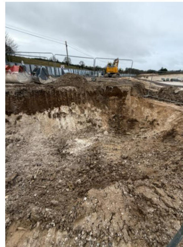
Deepened Trench 2 looking north
