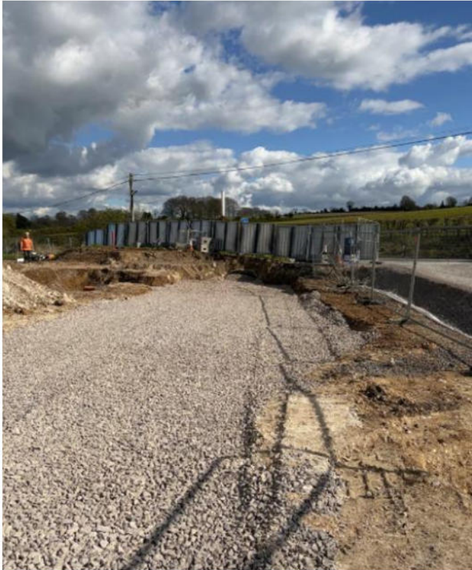
Backfilled Trenches looking south
