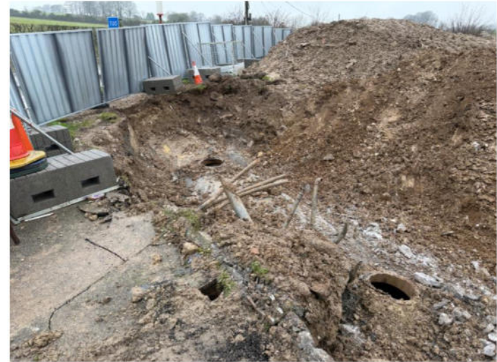
Breaking out of tanks in Trench 2
