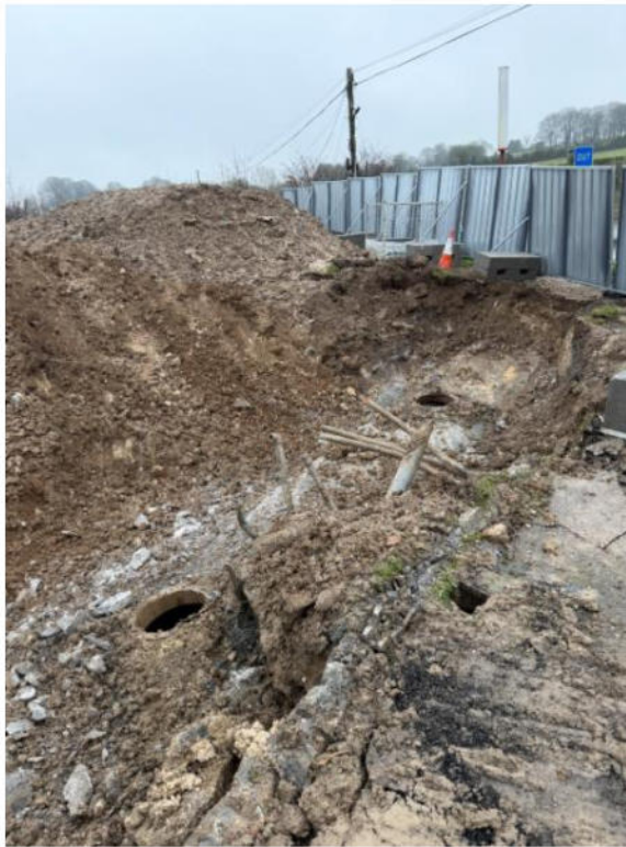
Breaking out of tanks in Trench 2
