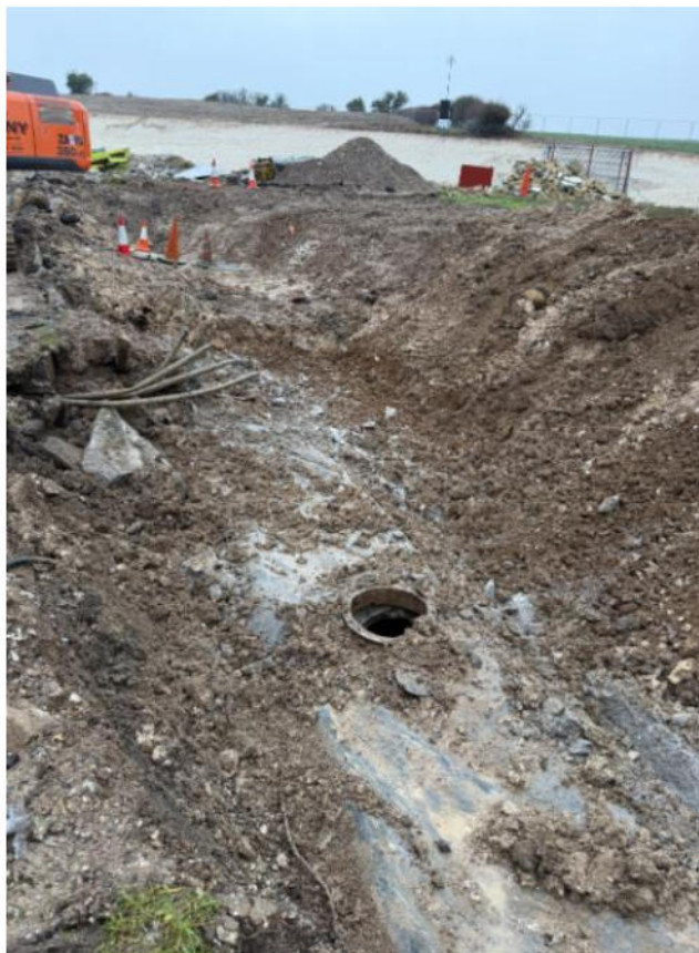
Breaking out of tanks in Trench 1
