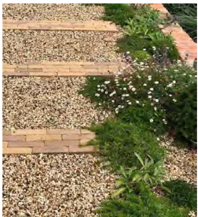
CLAY PAVERS ACT AS STEPPING STONES IN GRAVEL LEAD FROM SPA TO FUNCTION BUILDING
