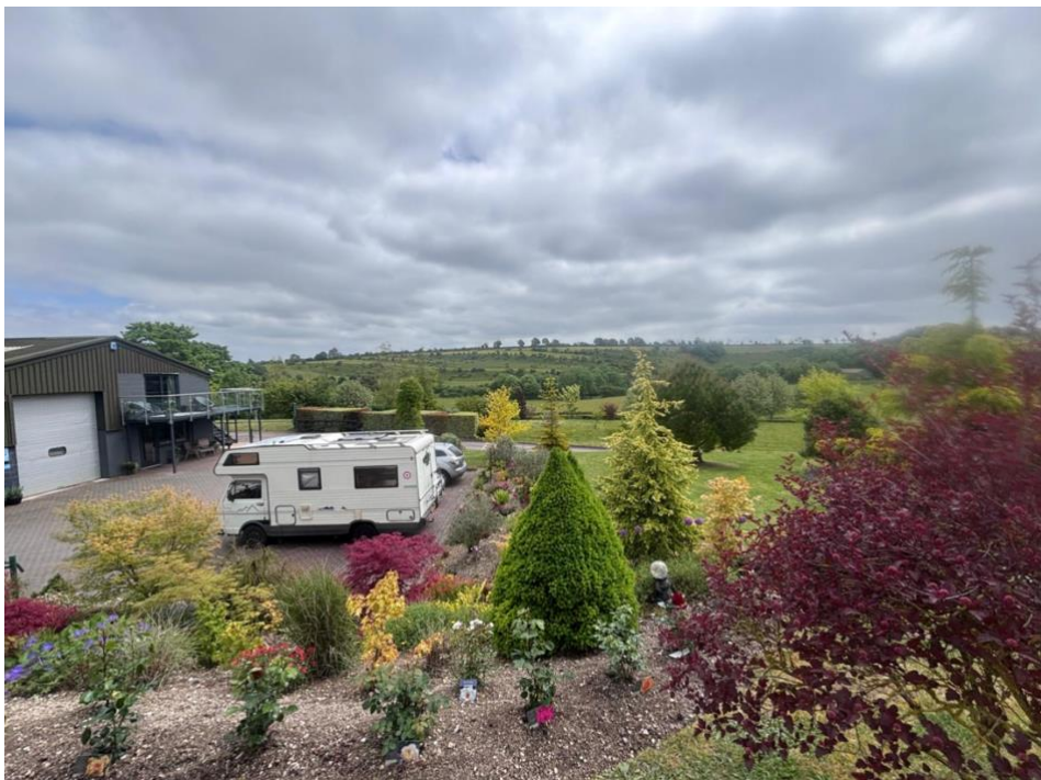
Figure 5: View from upper part of the garden back toward the workshop building, balcony and forecourt.
