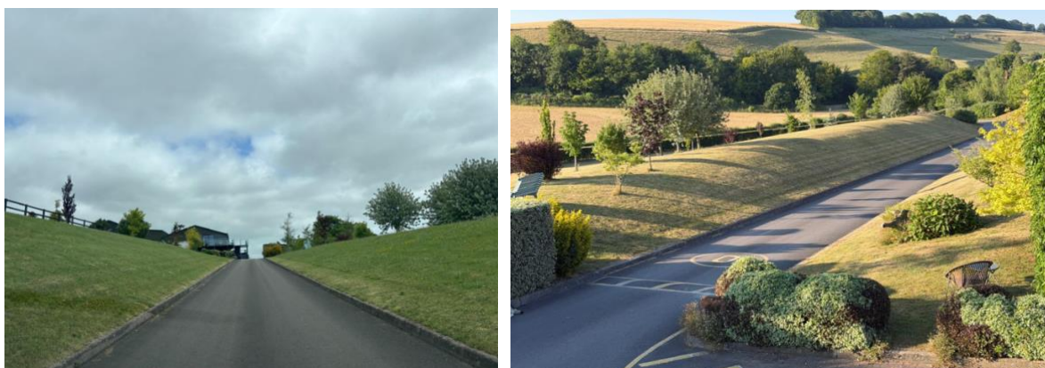
Figure 8: Views on the approach, to and from Coombe Down Farm, showing the existing engineered site entrance and developed context.
