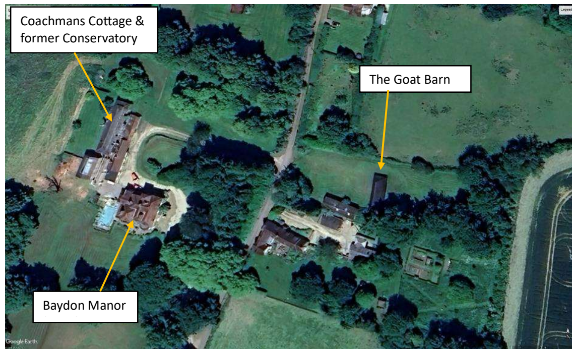
Aerial view of the Goat Barn and its context (Google Earth)
