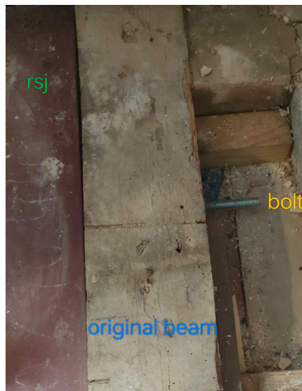
PHOTO: BEAM INSTALLATION - viewed beneath floorboards from above
