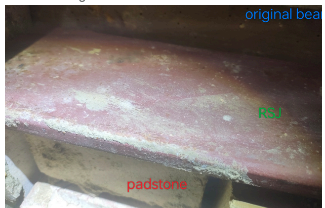
PHOTO: installed structure (viewed from First Floor floor)
