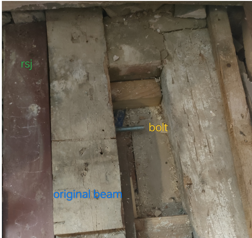
Photo: view of top of structure beneath floorboards from First Floor - new steel channel bolted to existing timber beam.
