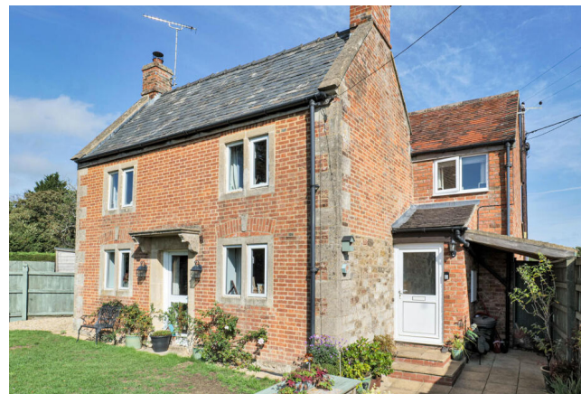
PHOTO: Building frontage
