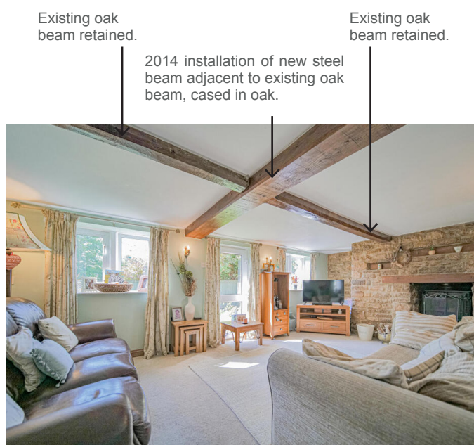
PHOTO: BEAM THROUGH LIVING ROOM
