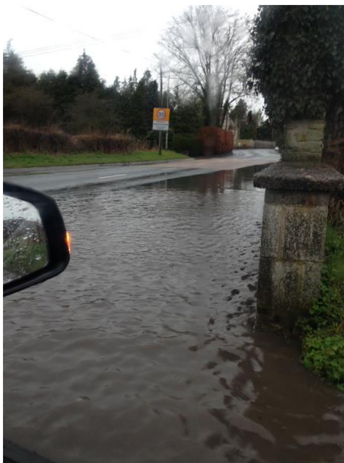
Figure 1 – Surface water flooding across Boreham Road
