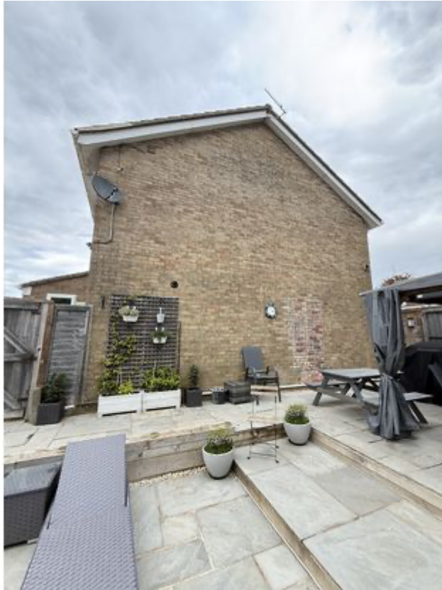
Figure 5 – Gable end (south) elevation viewed from side garden, showing extent of blank gable wall and existing patio
