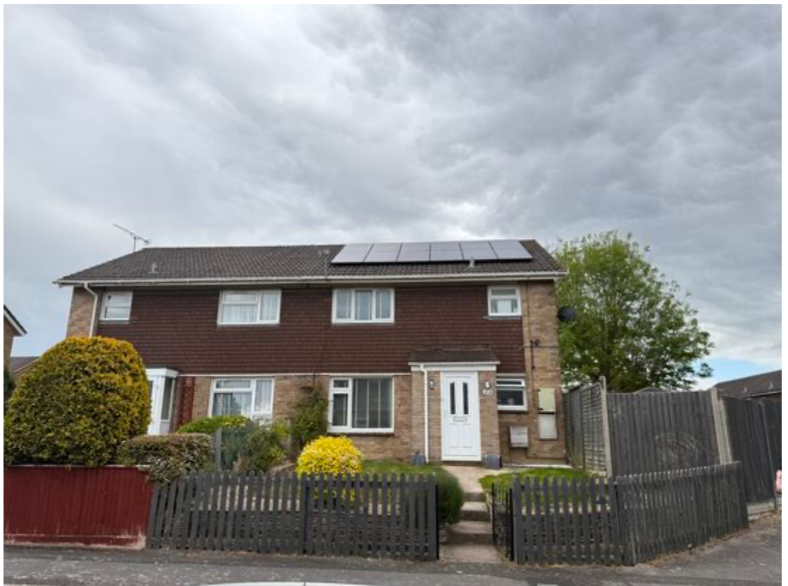
Figure 2 – Front elevation viewed from Orchard Way, showing wider street context and neighbouring property
