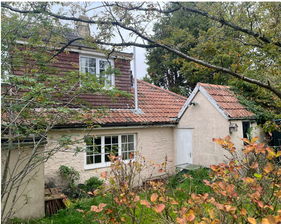
View of Rear [East] Elevation of Existing Dwelling House
