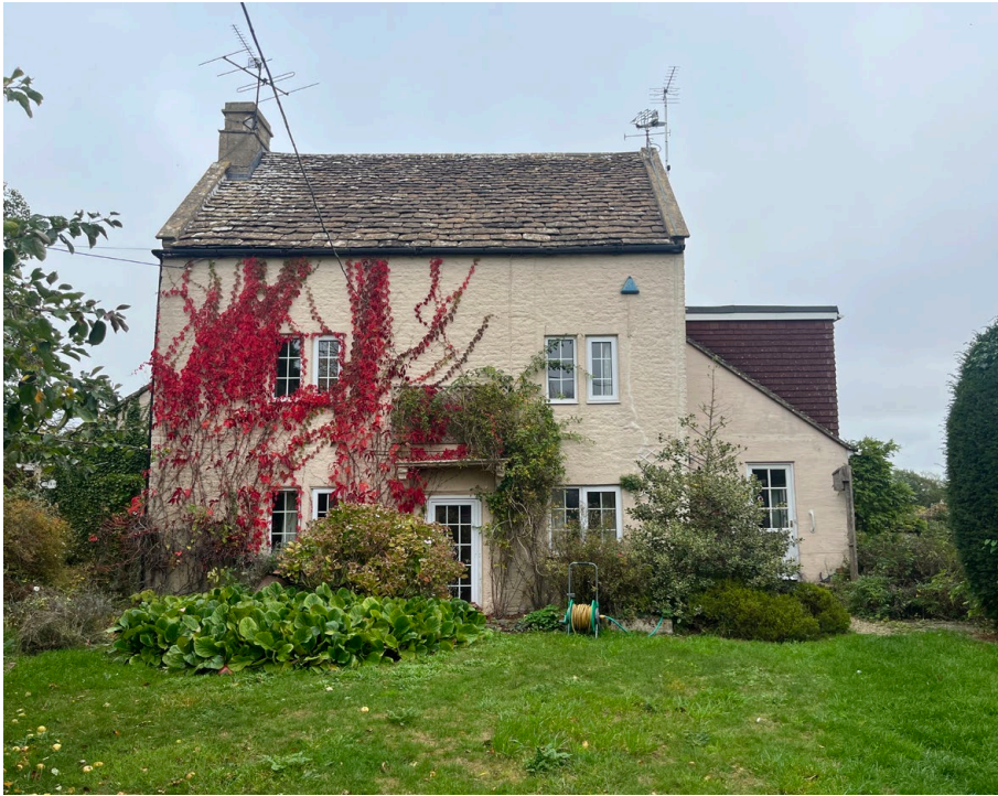
View of Front [West] Principal Elevation of Existing Dwelling House
