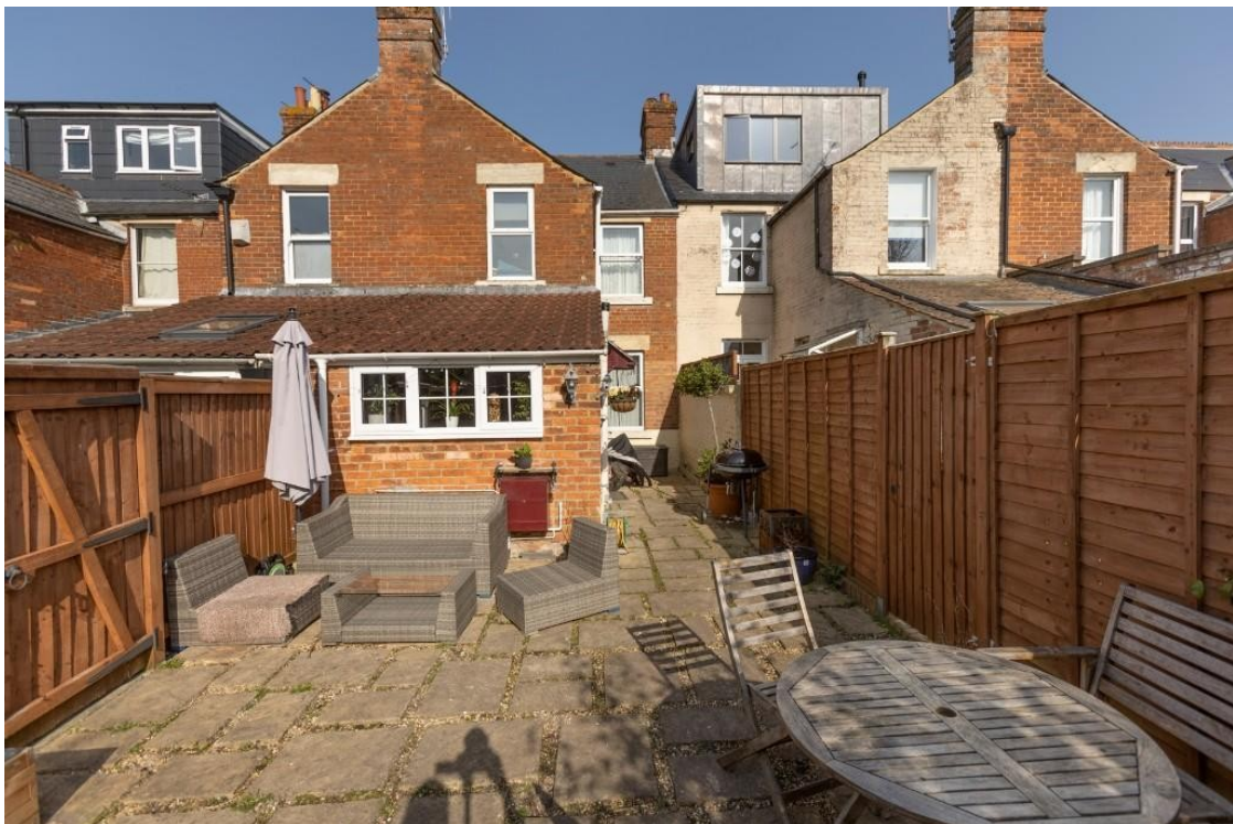
Bottom: Rear aspect as viewed from rear garden showing gable ended outrigger and neighbouring dormers.
