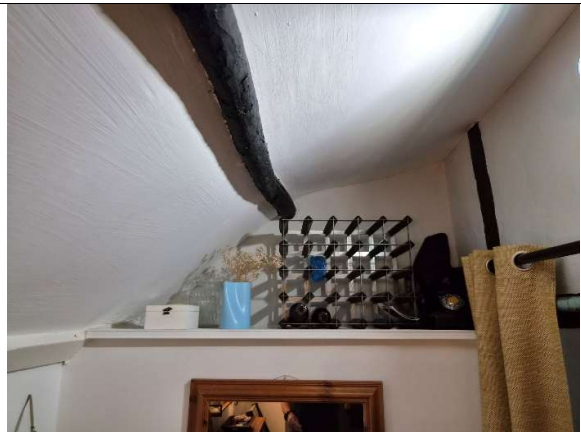
4. MDF shelf above wall, where masonry removed. Note purlin
