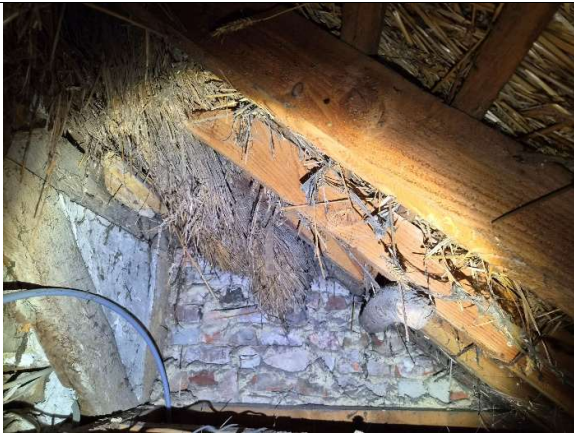
1. View of wall as viewed from roof space
