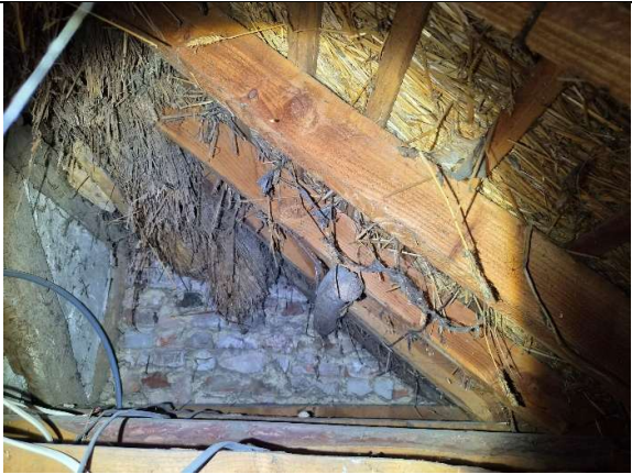
5. View of modern rafters and ceiling joists above shower room.
