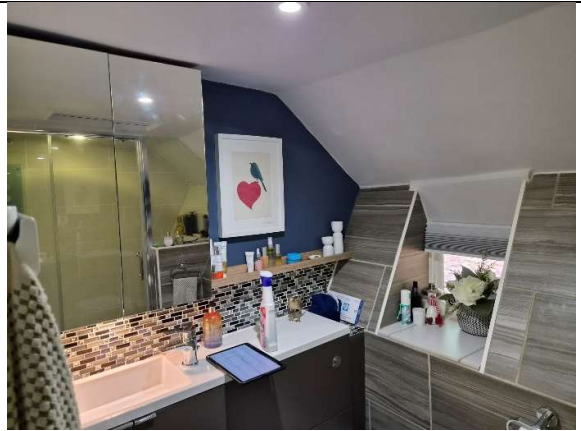
6. View of wall from shower room side
