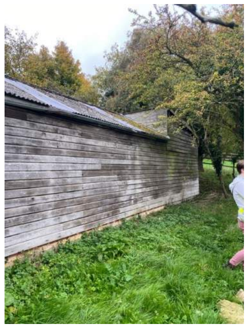
Photo 4 – Main West Elevation, South End
