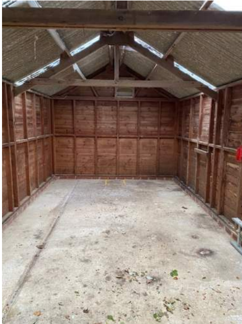
Photo 1 – Structural elements with exposed interior, main wing looking south.
