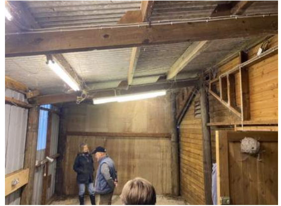
Photo 2 – Structural elements with exposed interior, south wing
