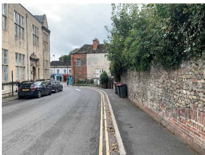
S facing view along the eastern site boundary
