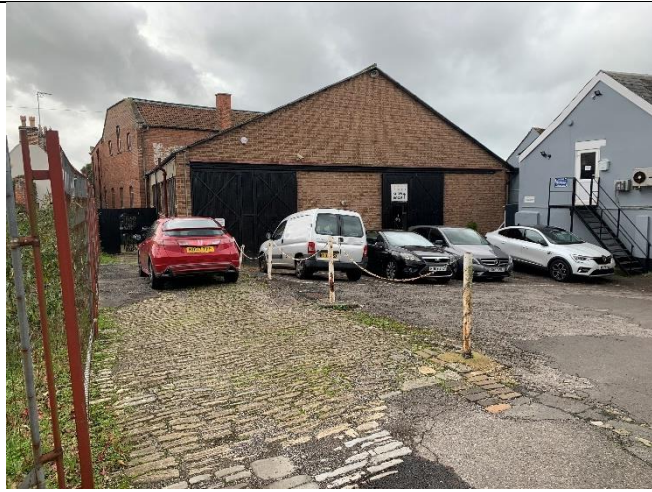
S facing view along the western site boundary
