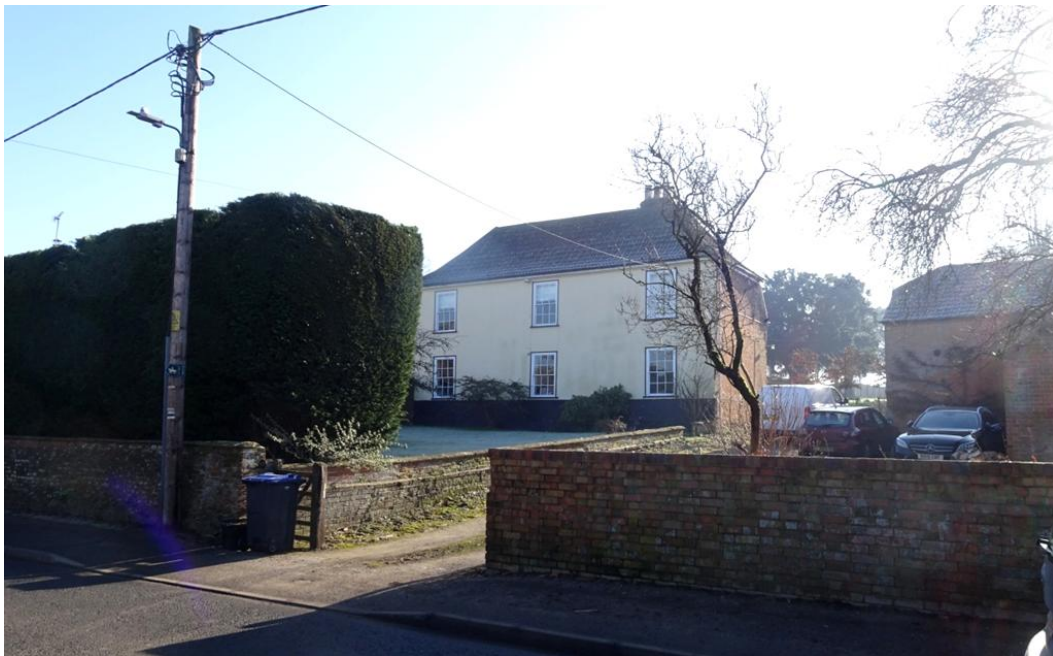
Photo 2. Manor Farm House from High Street, with the outbuildings on the extreme right
