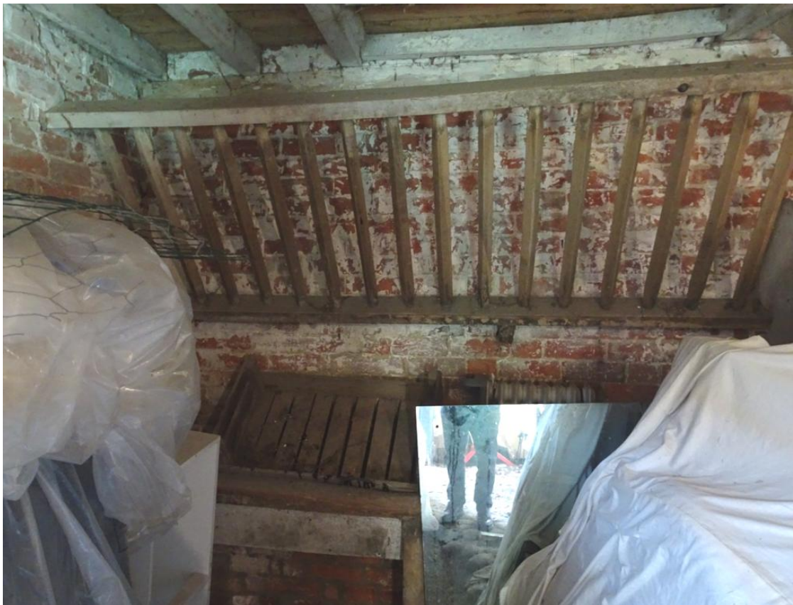
Photo 3. The hayrack and manger (partly obscured by a mirror)
