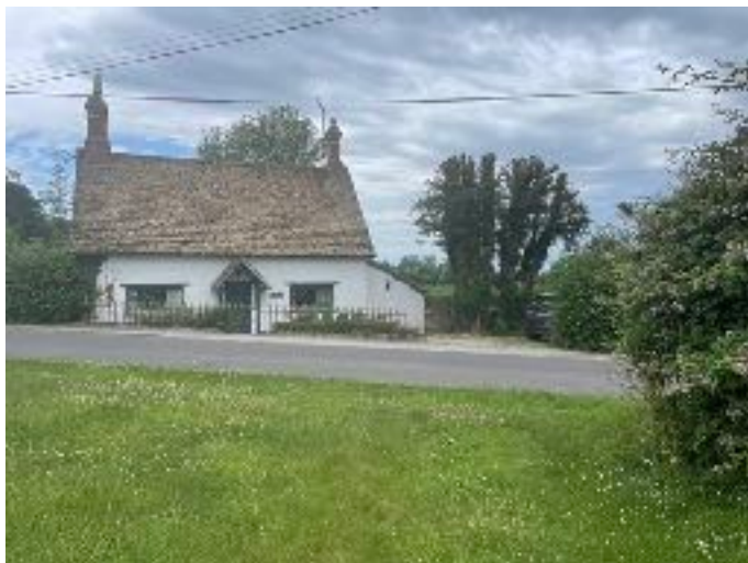
View of number 47 from proposed new vehicle entrance - note position/height of windows in relation to road.
