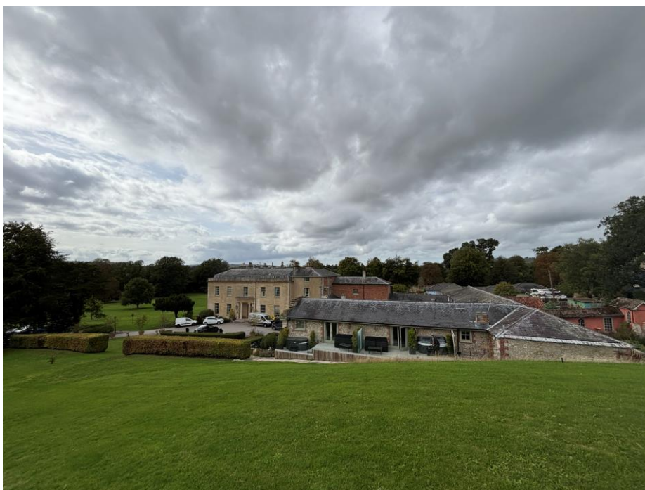
Fig.14 Bishopstrow House Hotel and Spa as seen from the higher ground of the bowl barrow to the east; the hotel has a well-treed and verdant backdrop
