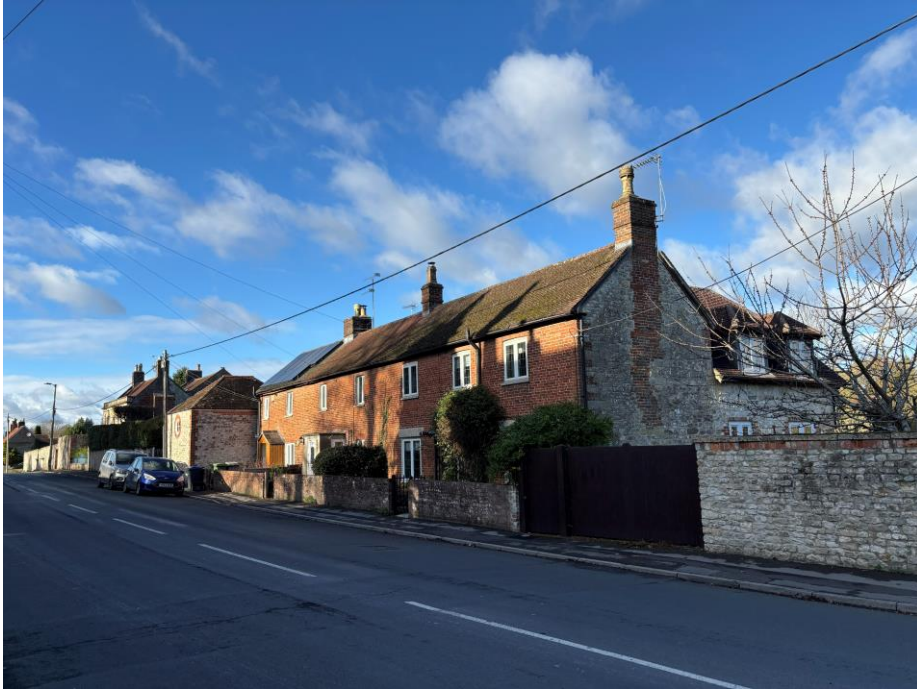
Fig.22 Nos. 209-215 Boreham Road
