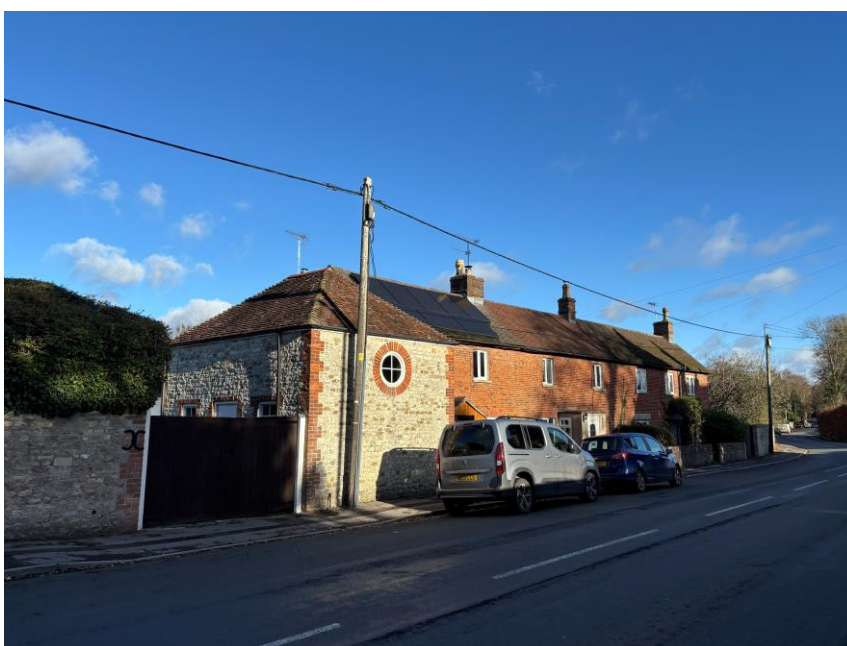
Fig.19 Stable building and adjacent terrace of brick cottages
