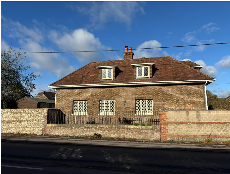
Fig.23 No. 215a Boreham Road (the old smithy)
