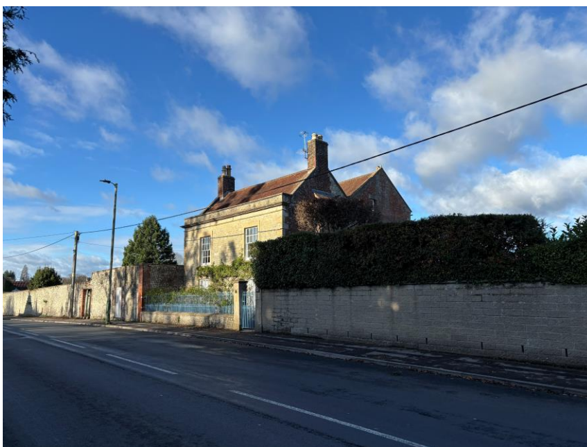
Fig.18 The Cotes and high stone boundary walls to either side
