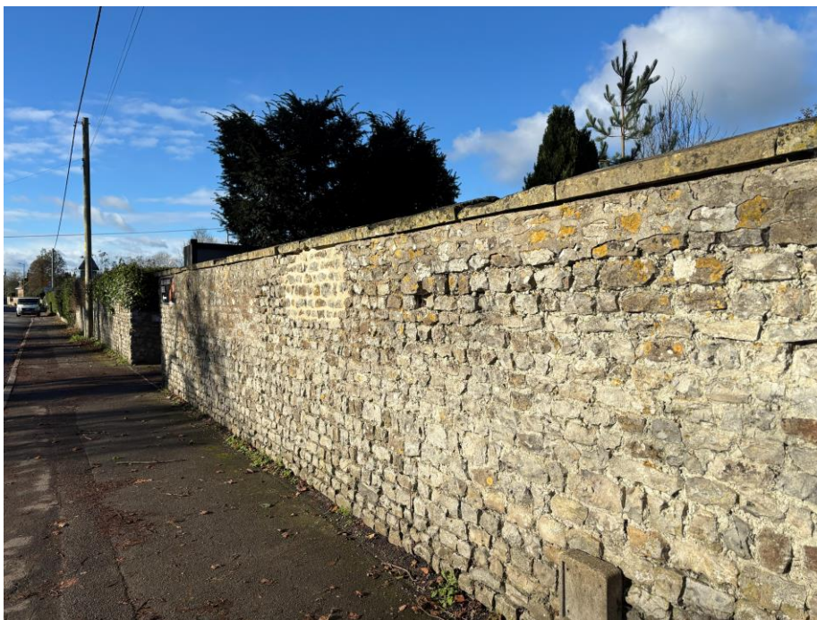
Fig.13 High stone boundary wall by the road to the east of Home Farm Lane
