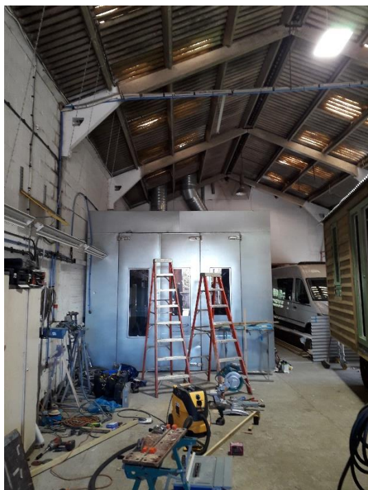
4: Spray booth inside building unit (Salisbury site)
