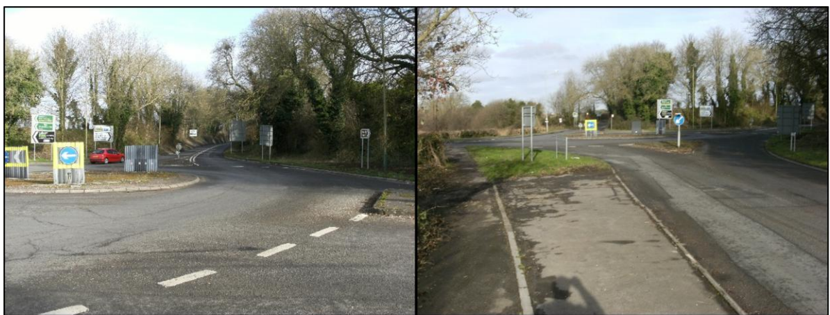
Plate 4.1 – A30/A338/Church Road Roundabout
