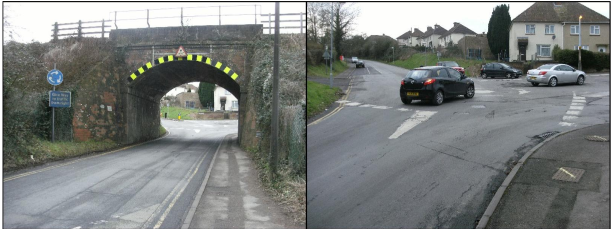
Plate 4.2 – Bourne Avenue / Laverstock Road Mini-Roundabout
