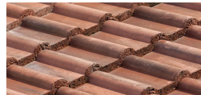
Roof – Double Roman tiles
