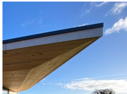
Walls/ Roof – Cedar Fascia/ Soffit detail
