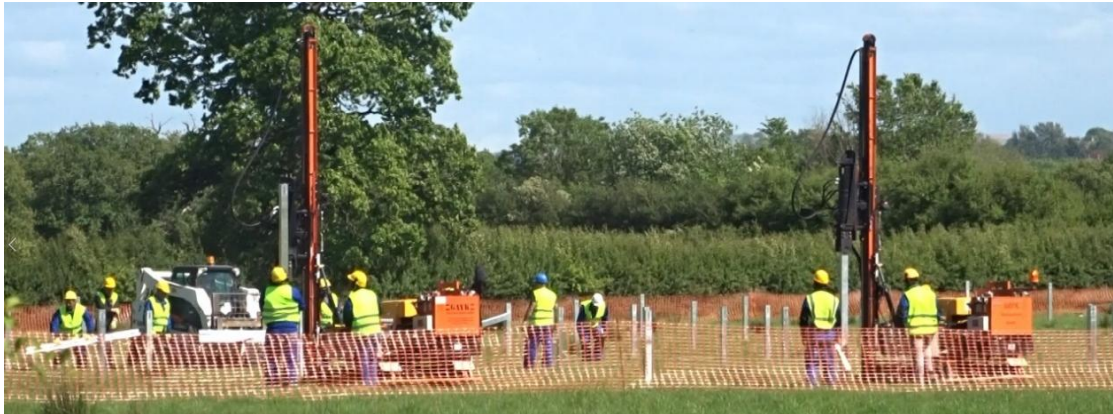
Photo 2: Posts Being Installed
