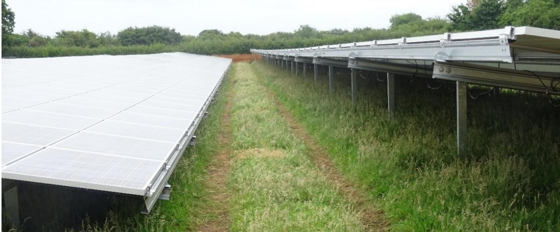
Photo 5: After Panels Bolted-On
