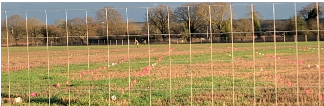
Photo 1: Marking Out in Progress
