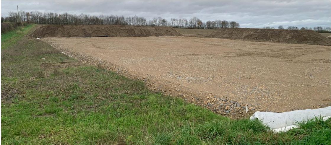
Photo 8: Example of a Construction Compound (this was for a water pipeline)
