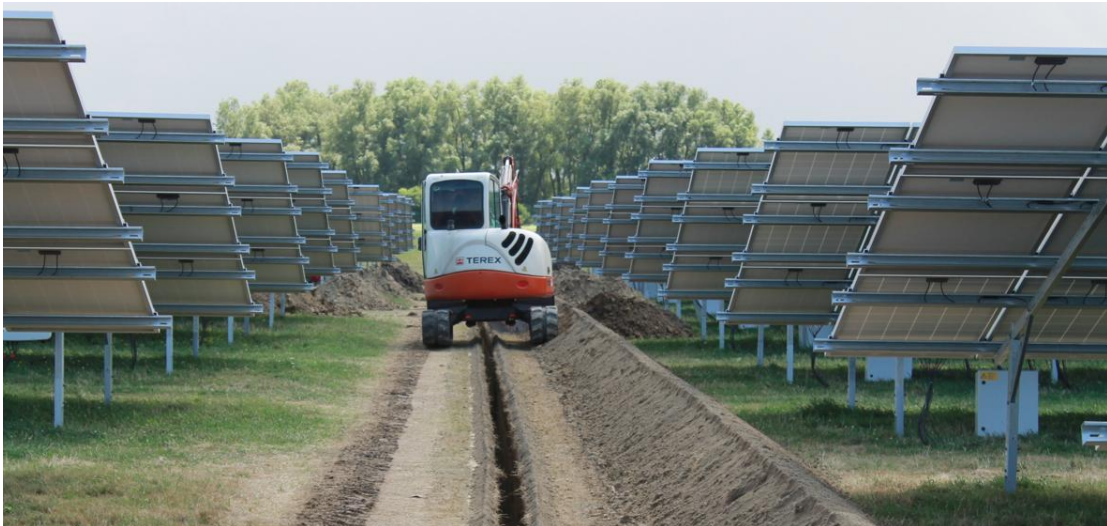
Photo 6: Trenching in Progress
