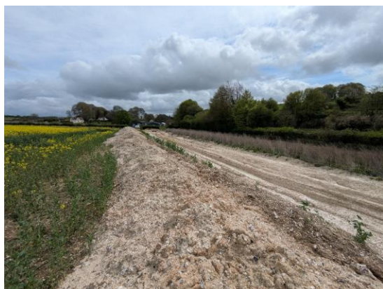
Figure 4.5. Western extent of parcel A4
