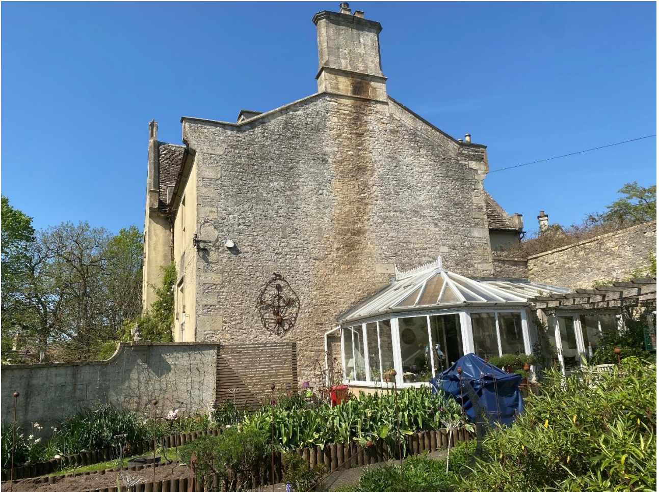
Figure 8 – Angled view of the east elevation, including the existing conservatory.
