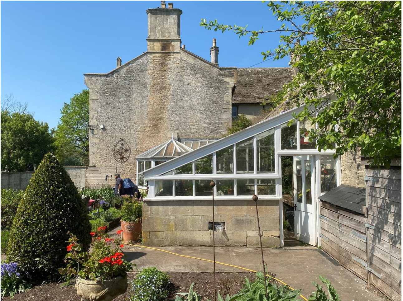
Figure 7 – The Old Rectory – east gable elevation with greenhouse and conservatory.
