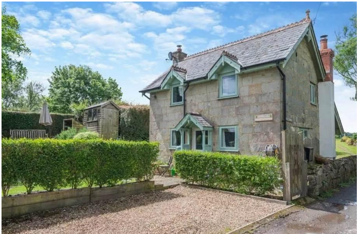
Fig 3.2.4: Principal elevation before the garden room
