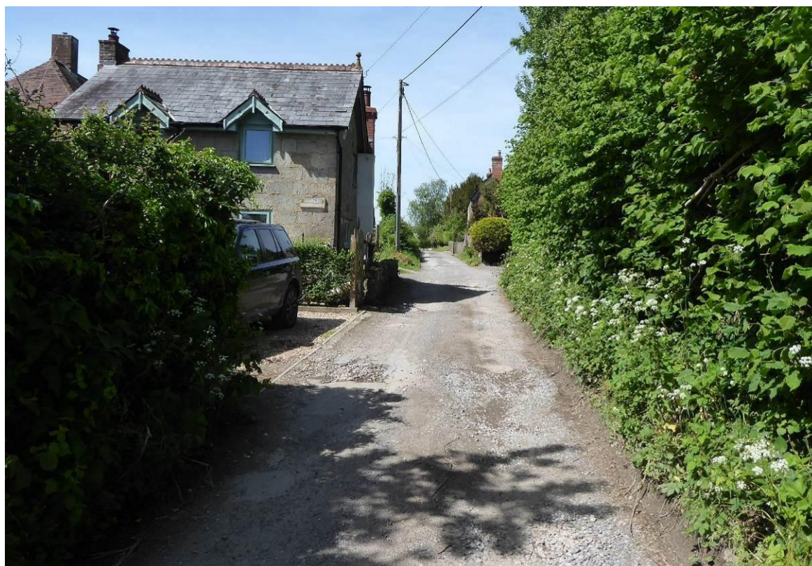
Fig 3.4: The garden room is not visible when approaching the site from the east
