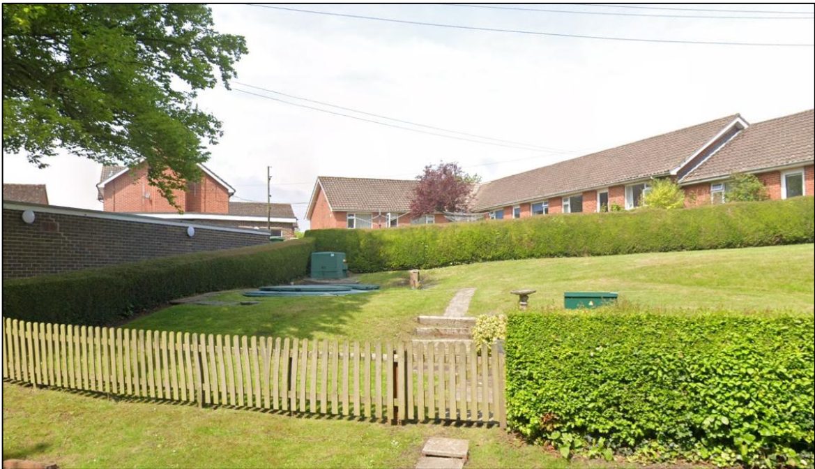
Figure 2: Google Street View extract showing the existing PTP
