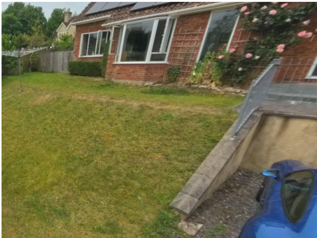
Figure 2 Looking north to show existing lawn and retaining wall
