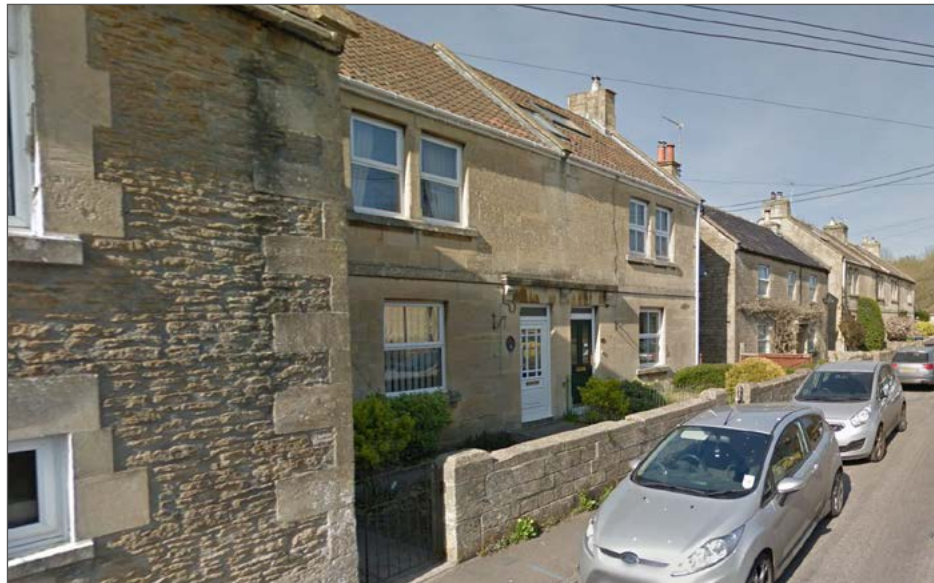
Period properties on Westwells Roads, Westwells.
