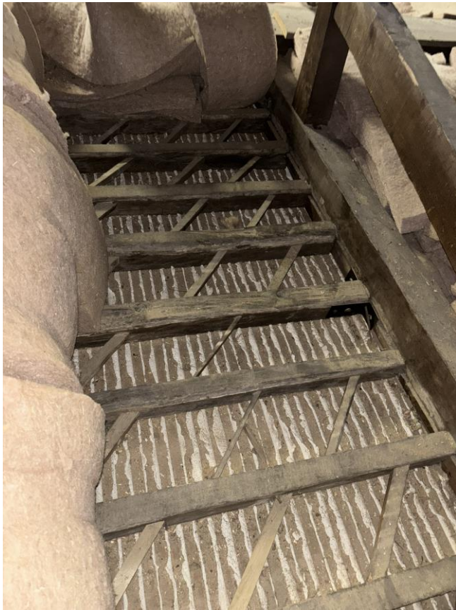
013 Area of medium risk area is all well keyed and seems secure.
