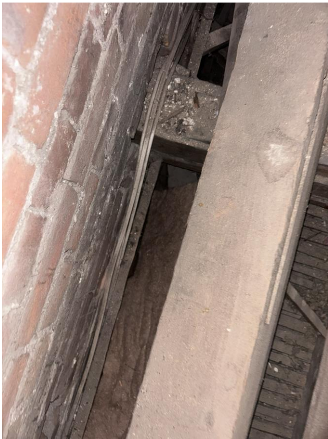
019 Area behind cornices evidence of insulation.
