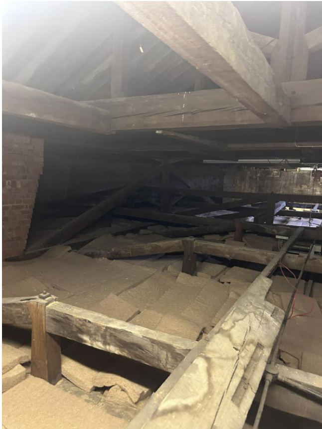
017 Overview of loft space.
