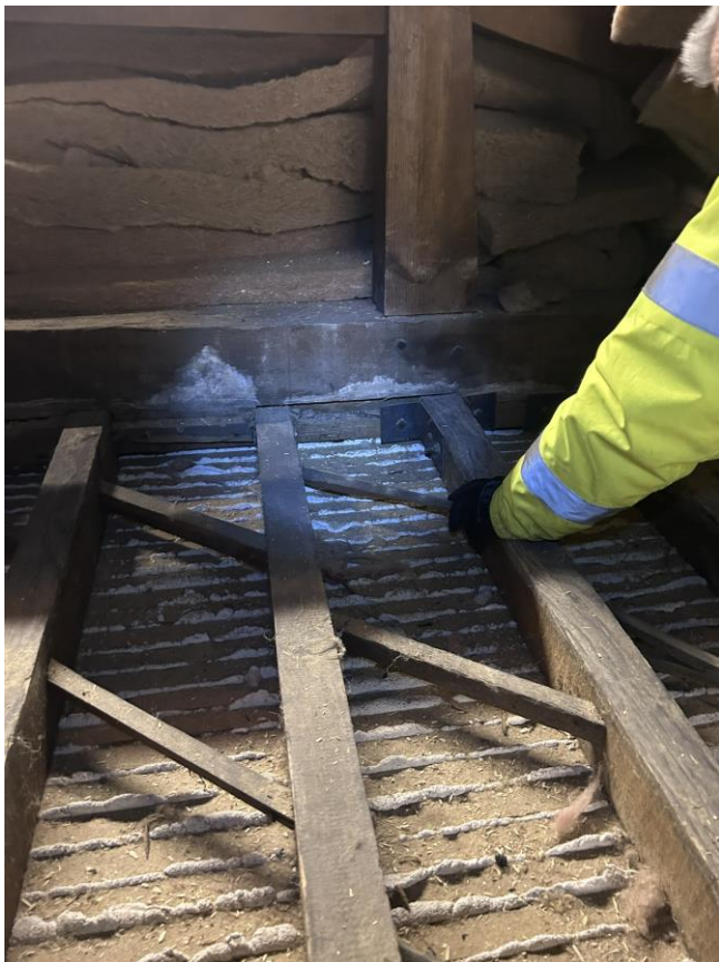
020 Low risk area appears to be well keyed and intact and secure.
