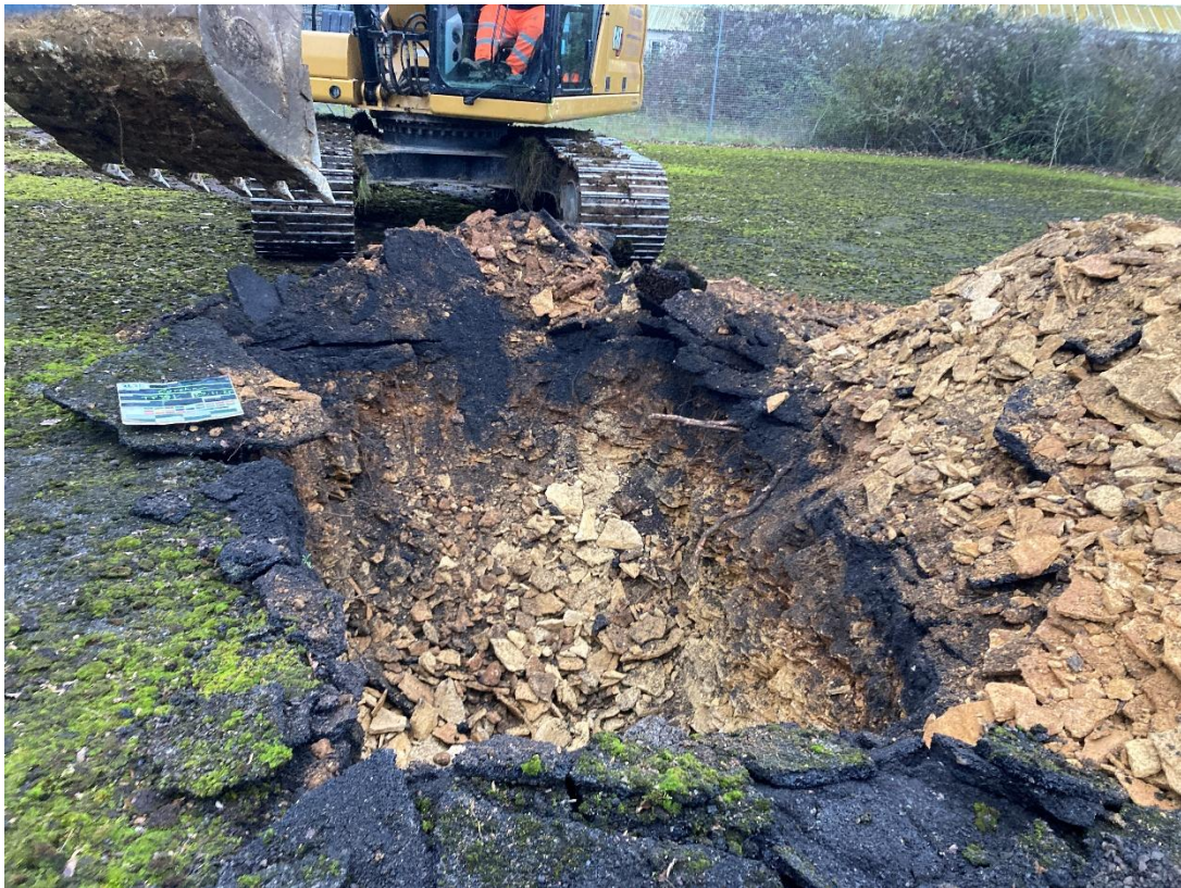
Photograph 1 – Side view of TP301 and its arisings, excavated to 3.70m bgl.
