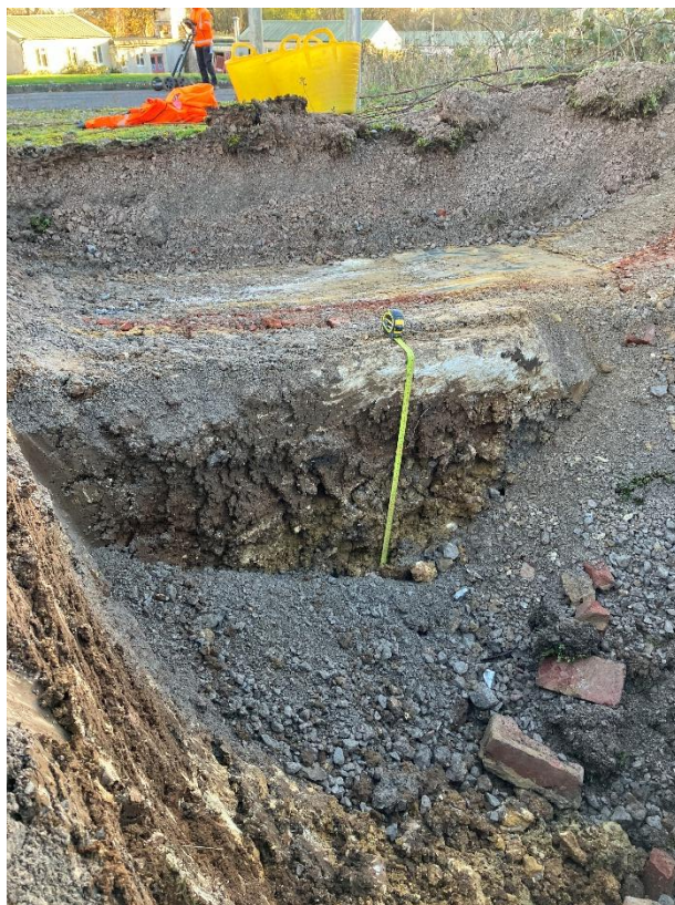
Photograph 4 – Side view of TP304 and a concrete footing, excavated to 1.50m bgl.
