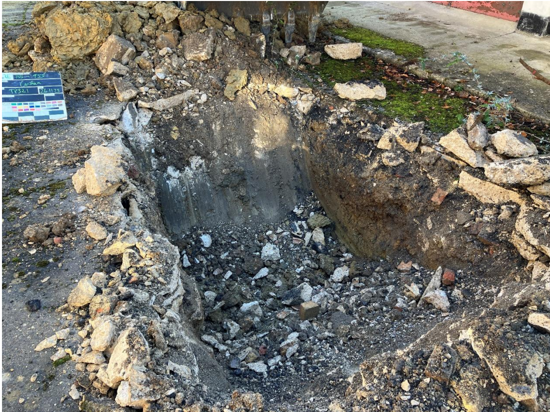
Photograph 17 – Side view of TP321 and its arisings, excavated to 1.20m bgl.
