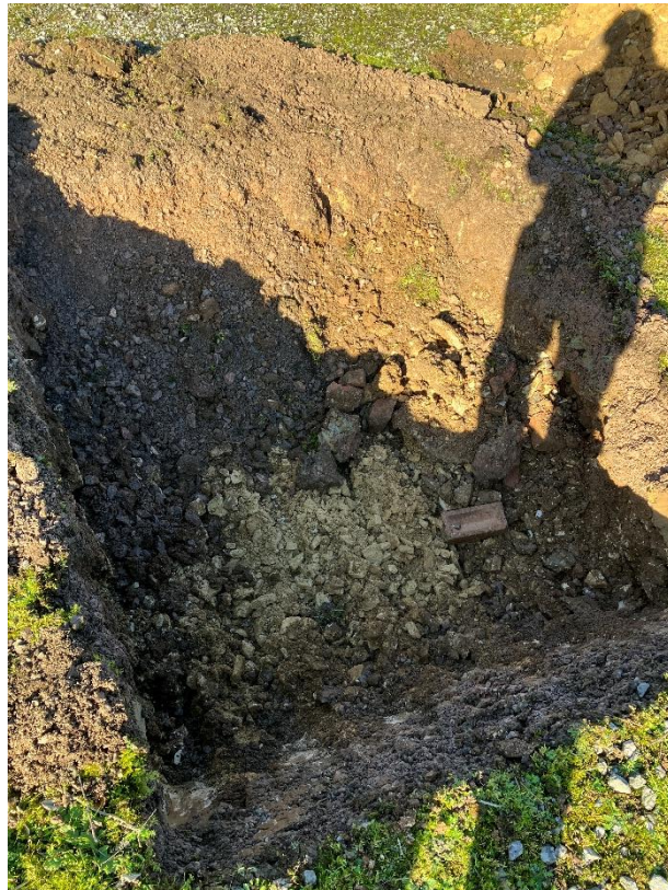
Photograph 3 – Side view of TP303 and its arisings, excavated to 0.90m bgl.
