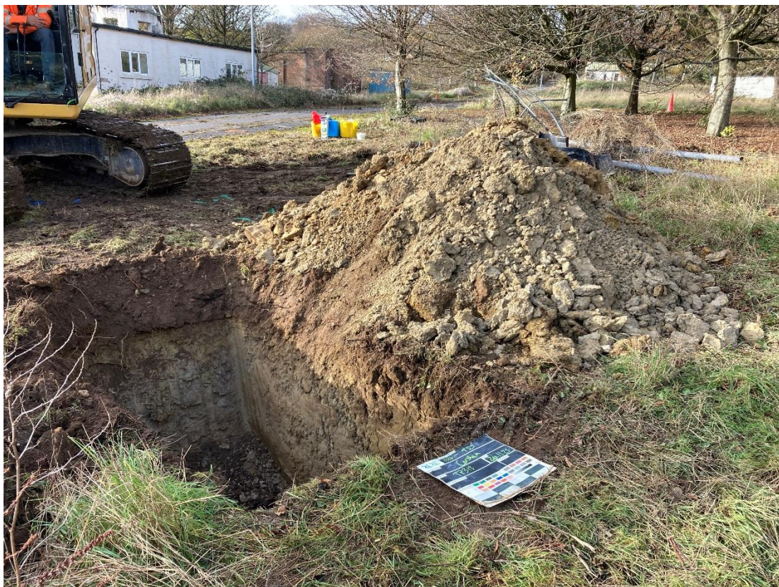
Photograph 14 – Side view of TP313 and its arisings, excavated to 1.90m bgl.
