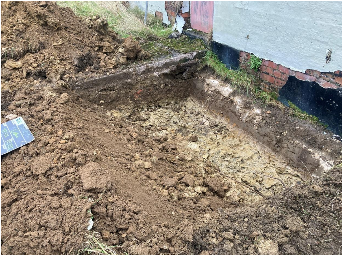
Photograph 22 – Side view of TP328 and its arisings, excavated to 0.80m bgl.
