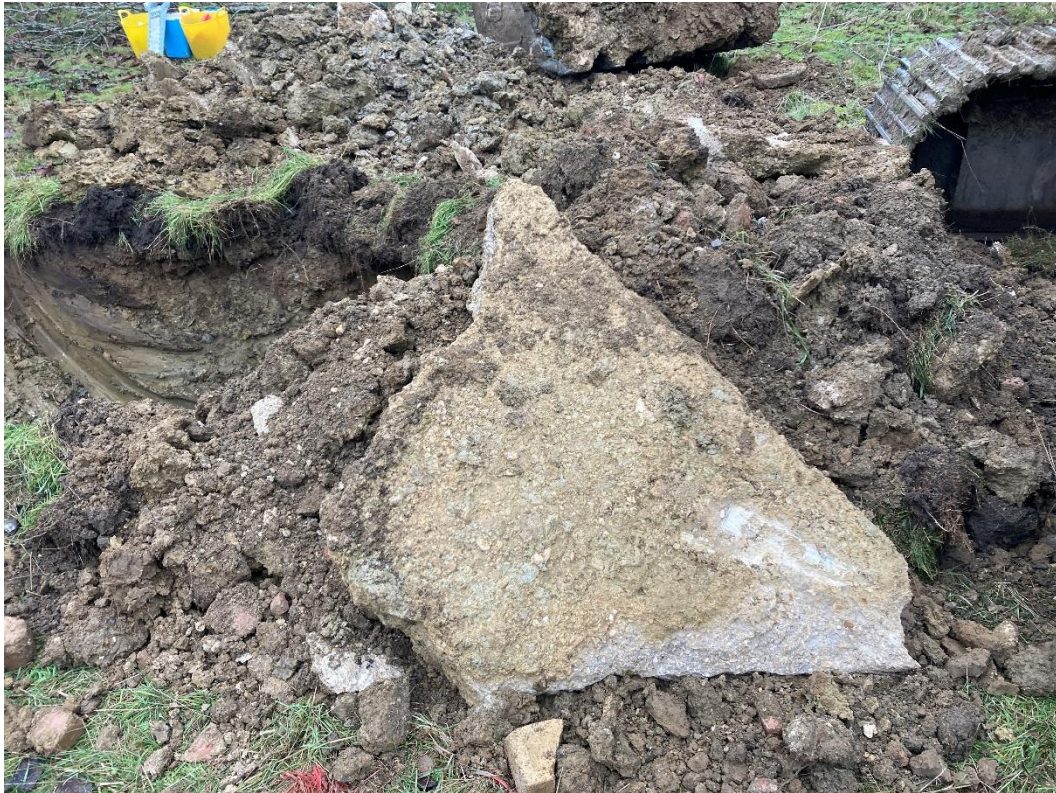
Photograph 9 – Concrete slab excavated from TP308.
