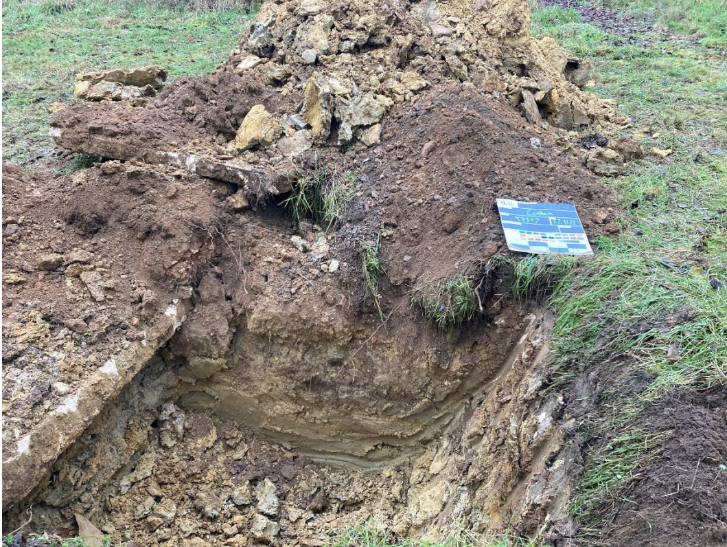
Photograph 7 – Side view of TP307 and its arisings, excavated to 1.40m bgl.
