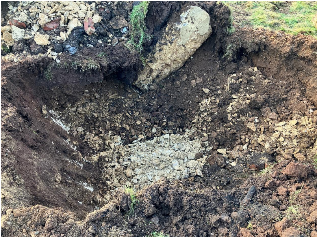
Photograph 2 – Side view of TP302 and its arisings, excavated to 1.00m bgl.
