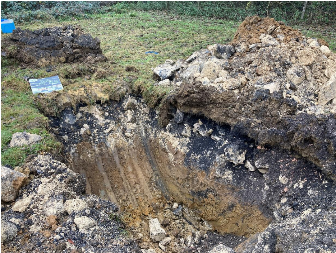
Photograph 6 – Side view of TP306 and its arisings, excavated to 1.80m bgl.
