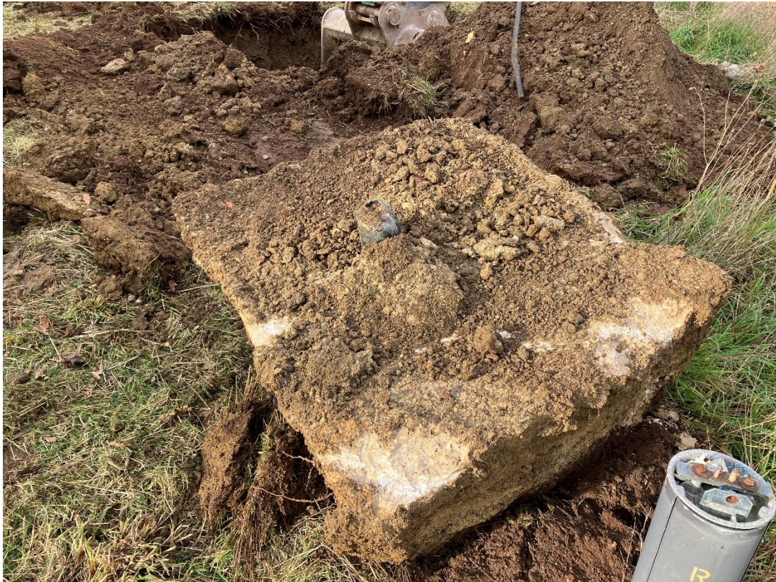
Photograph 13 – Concrete footing found in of TP312.
