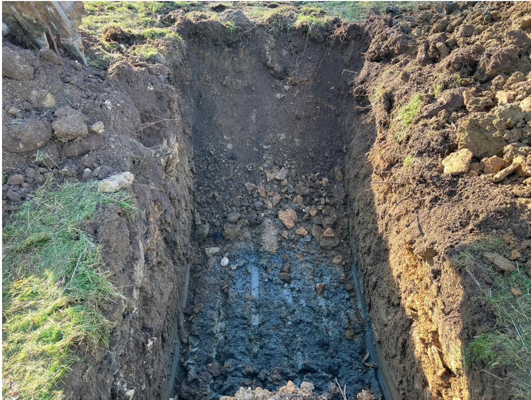
Photograph 11 – Side view of TP311 and its arisings, excavated to 1.63m bgl.
