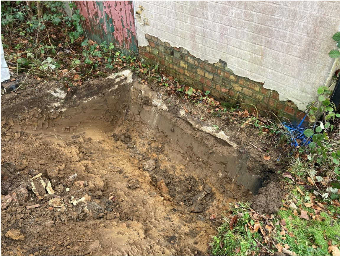
Photograph 23 – Side view of TP329 and its arisings, excavated to 0.84m bgl.
