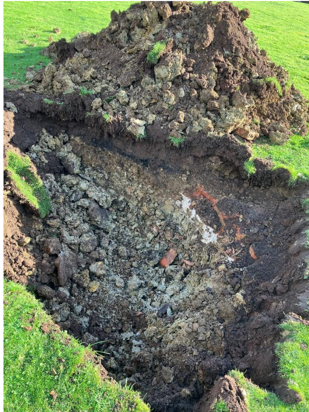
Photograph 5 – Side view of TP305 and its arisings, excavated to 1.00m bgl.
