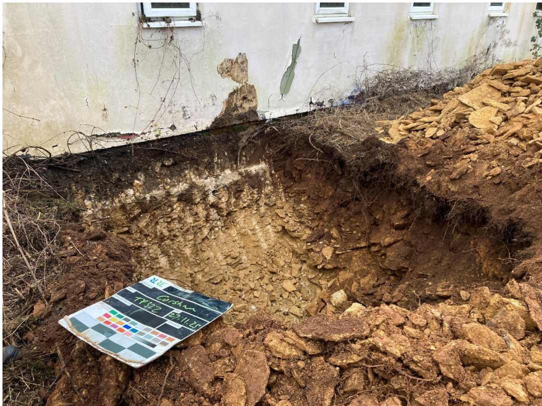
Photograph 18 – Side view of TP322 and its arisings, excavated to 1.60m bgl.
