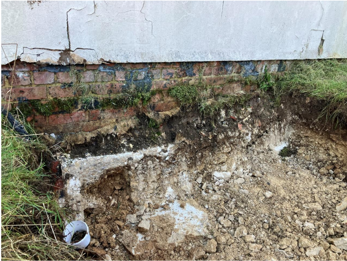
Photograph 19 – Side view of TP324, excavated to 0.70m bgl.
