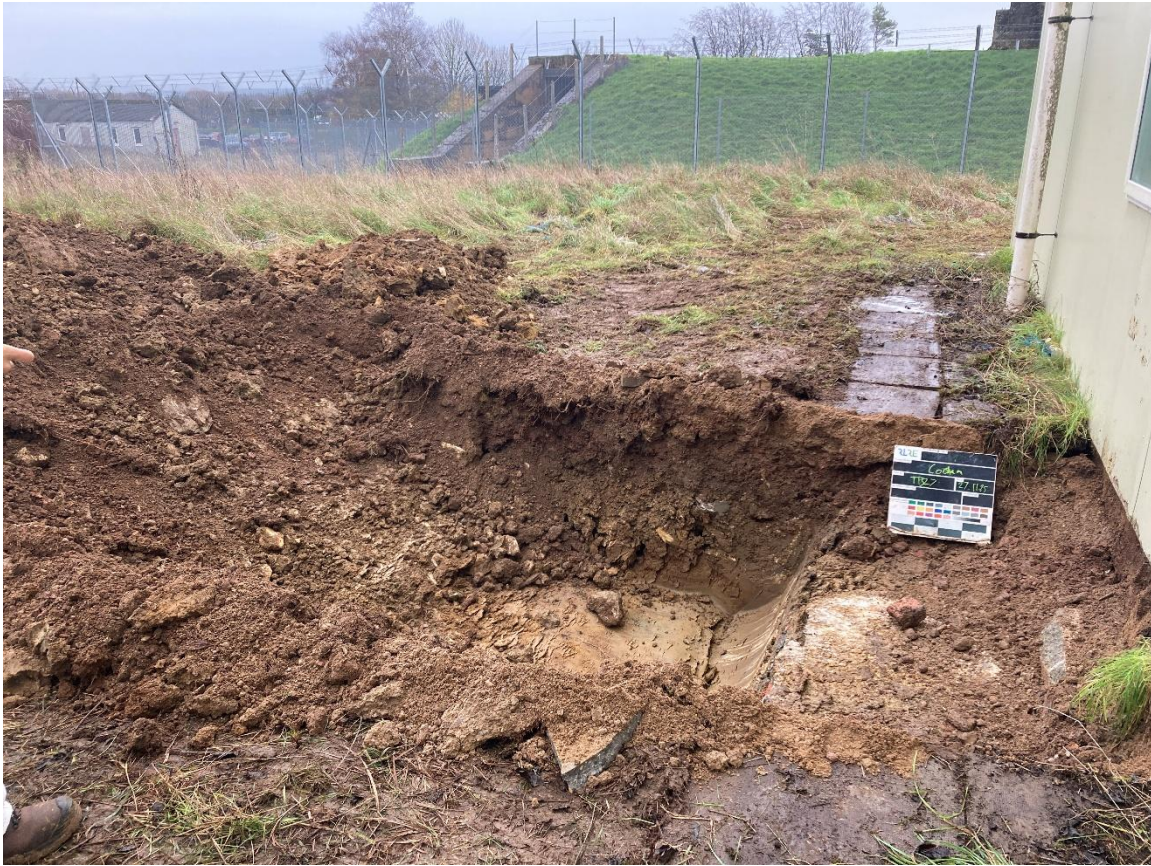
Photograph 21 – Side view of TP327 and its arisings, excavated to 1.00m bgl.
