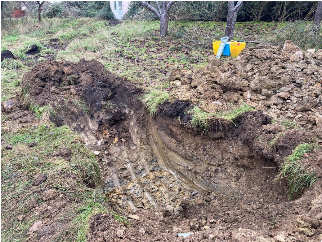
Photograph 8 – Side view of TP308 and its arisings, excavated to 1.300m bgl.
