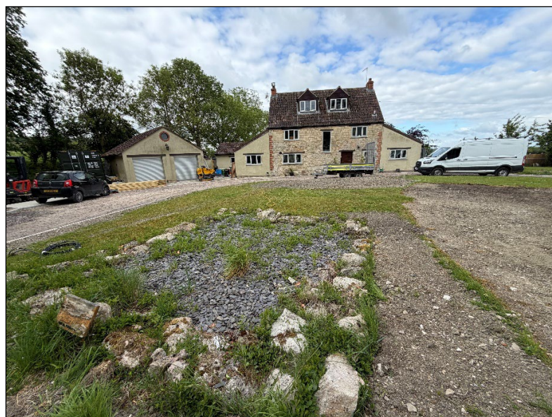
Image 10: Excavation area marked by stone boundary – Bincknoll cottage in background
