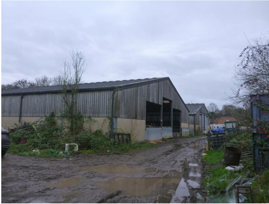
Fig 4: The barns have block walls and slatted wooden cladding.
