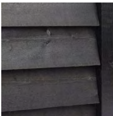
Dark stained horizontal weatherboard cladding
