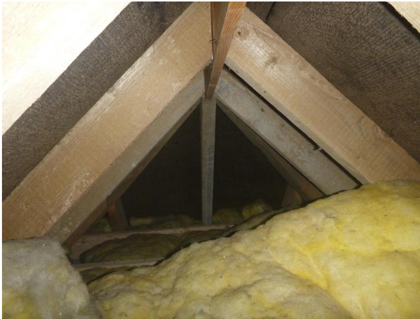
Fig 7: The small areas of loft space above the dormer windows were accessible.
