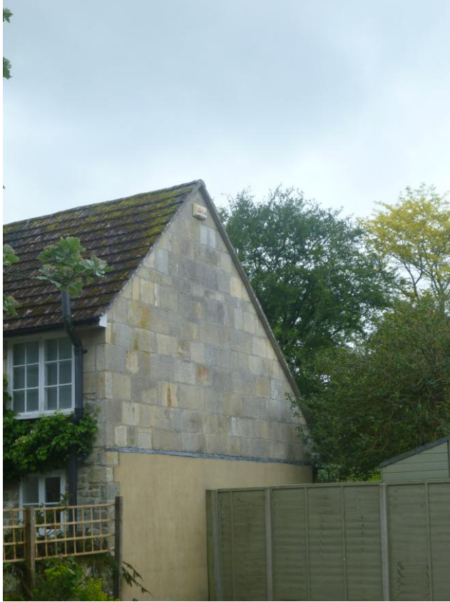
Fig 4: The mortar at the roof verges is in a good state of repair with none noted to be missing or damaged.
