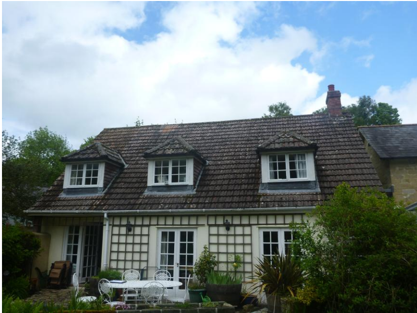
Fig 3: There is a catslide roof incorporating three dormer windows to the rear of Cleeve Cottage.
