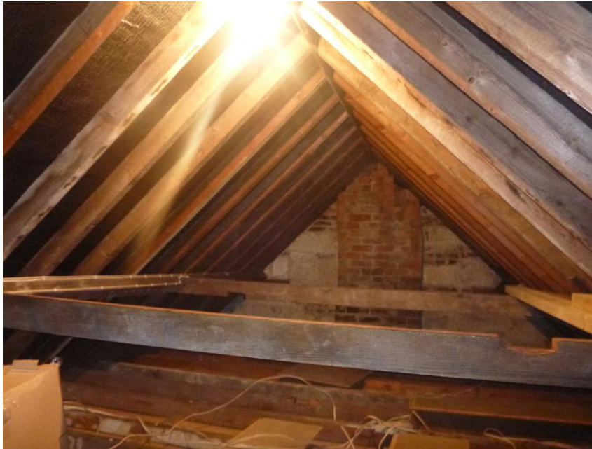
Fig 6: The roof is lined with bitumen felt and all areas of the loft space were accessible.
