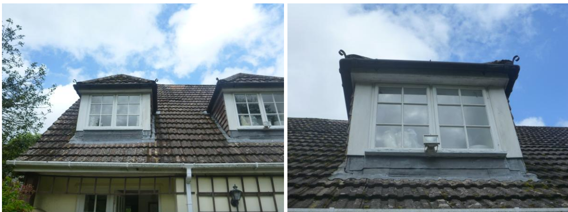
Fig 5: The dormer windows to the rear of the property are well sealed.
