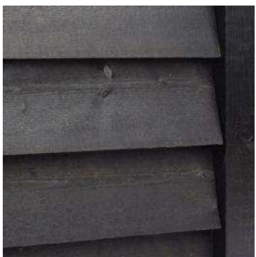
Dark stained horizontal weatherboard cladding
