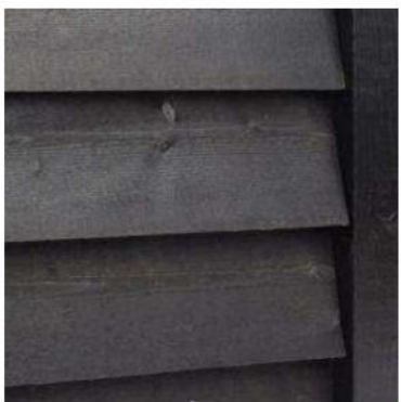
Dark stained horizontal weatherboard cladding
