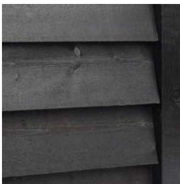
Dark stained horizontal weatherboard cladding
