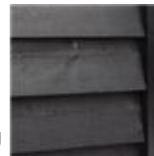
Dark stained horizontal weatherboard cladding
