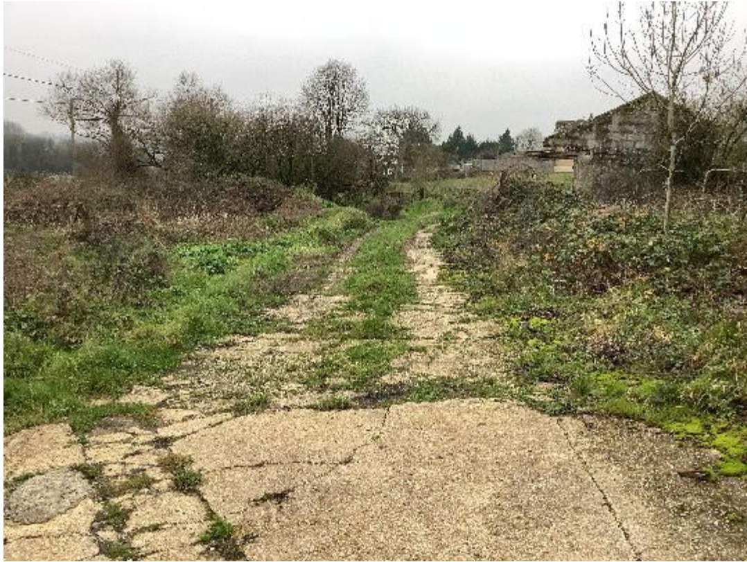
Main site – scrub, buildings and concrete habitats in south of site
