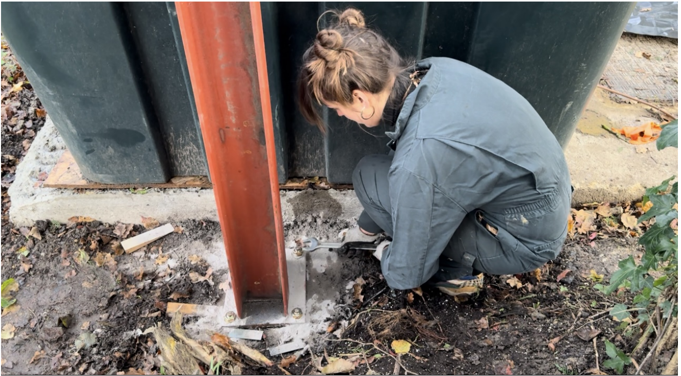
Installation photograph showing the fixed base of a steel post forming part of the replacement fence, set back from the former boundary position.
