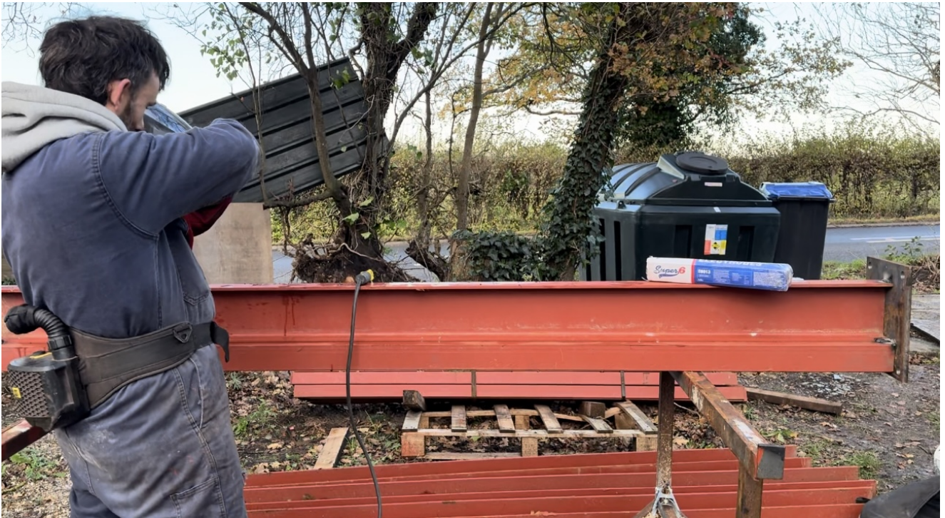
Construction photograph showing the fabrication of steel support members used to create the replacement fence.
