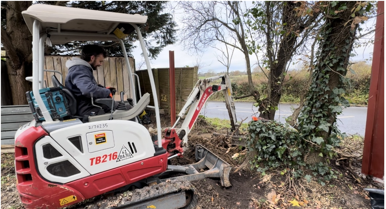
Construction photograph showing site works around the stepped-in boundary line and roadside edge.
