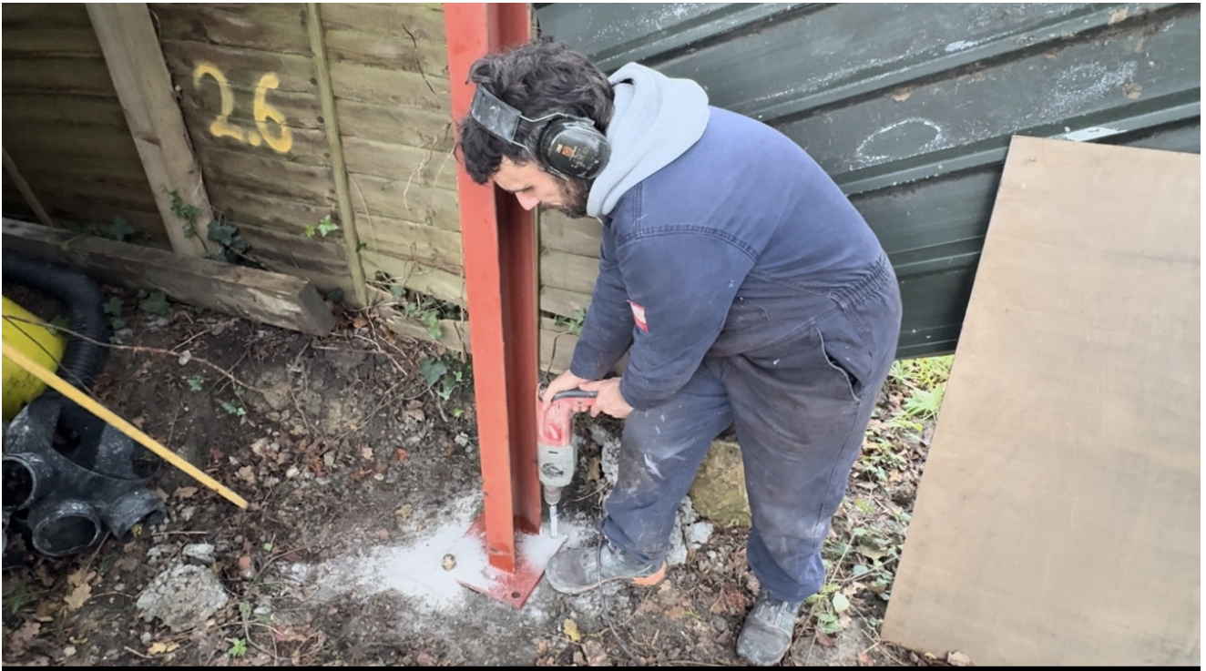
Installation photograph showing a steel post being set within the site as part of the replacement fence line.
