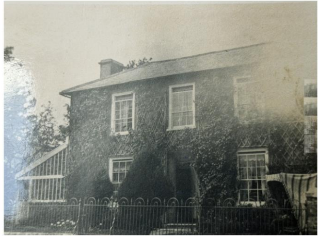
Figure 5: Early C20 photos of conservatory
