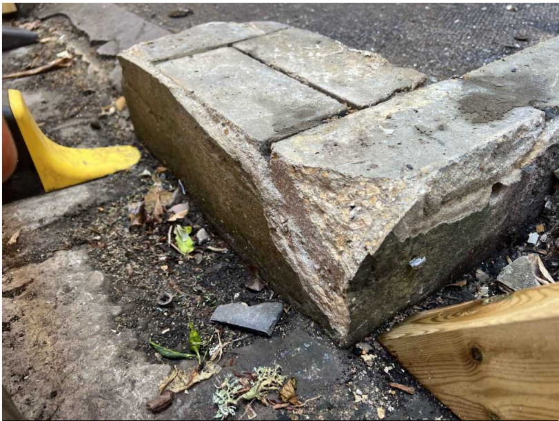
Pic.11 A section through the wall is exposed following removal of the damaged walling. A block at the right side quoin is broken, exposing its core, which is a concrete mix using a coarse natural stone aggregate. The external wall face to the front and around 150mm of the side has been rendered. (These are not stone faced blocks)
