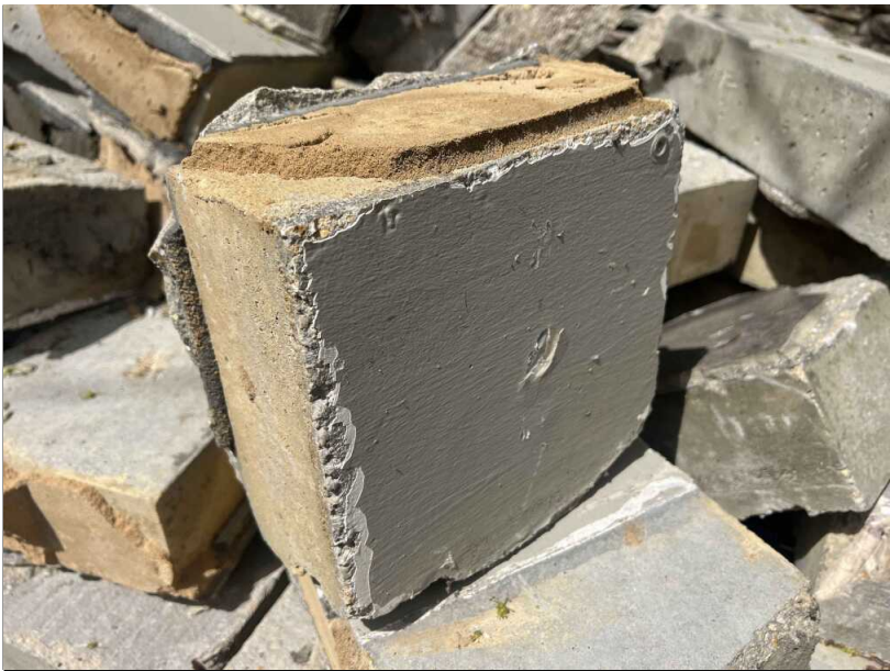
Pic.13 The internal face of the porch structure is a smooth plaster finish that has been coated with an oil based paint. The bed joint of the block appears to be a coloured cement mortar.
