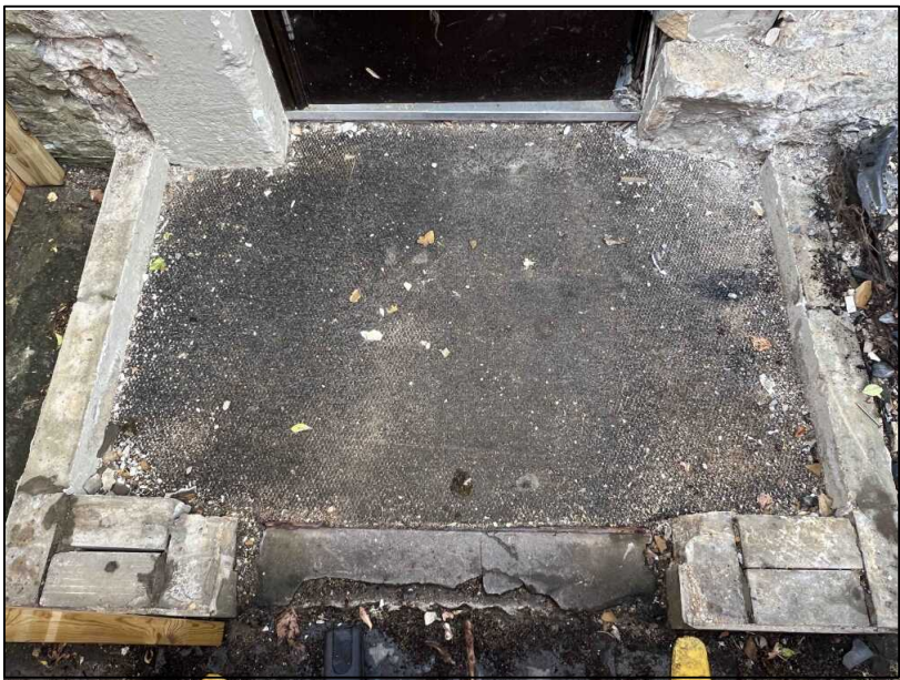
Pic.8 The substructure remains in-situ. The flank walls are 100 mm thick (plus the thickness of the cladding of approx 25mm). The front walls are 200 mm thick. The area has a covering of carpet over a screed and tile floor surface, sitting presumably above a concrete slab.
