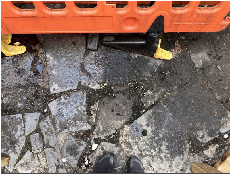
Pic.10 The ground area surrounding the porch structure is of random shaped natural stone laid upon and jointed in a cement mortar - 'crazy paving'. Excavation of the existing substructure will require some removal and reinstatement of this surfacing.
