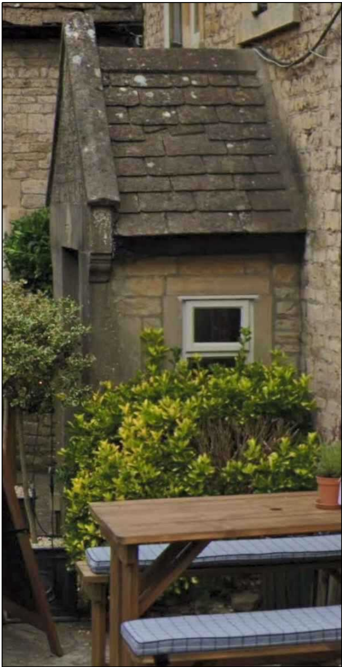
Pic.4 Further to the preceding image, - The Side elevation is shown here (Google Images 2025). Visible element in this image include: • Stone tiled roof covering in a diminishing gauge. • Fascia board at eaves • Side of profiled stone corbelled head • Random rubble effect side wall • Stone window opening surround • Casement window with top opening sash
