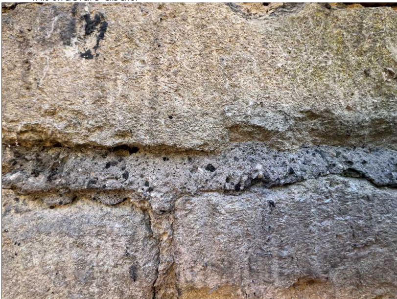
Pic.15 A close view of the mortar typical of the external elevation (there are other variants, but this is thought to be the most common). This is a lime based mortar with inclusions. This mortar is the one selected for the rebuilding works. Matching this mortar is thought to be straightforward.
