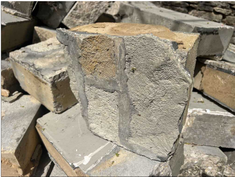
Pic.12 Some of the masonry from the demolition arisings was set aside. The external face of the 'random rubble effect stone' can be seen to be a two coat render that has been applied to the block walls, which has has some colouring added. The joints have been scribed and 'pointed' in a cement mortar. This finish is an attempt to replicate the appearance of the main building walls to which this structure abuts.
