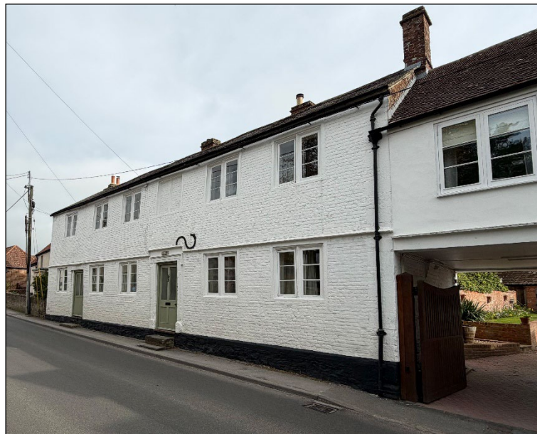
Image 21: Nos. 63 and 65 High Street, front elevation
