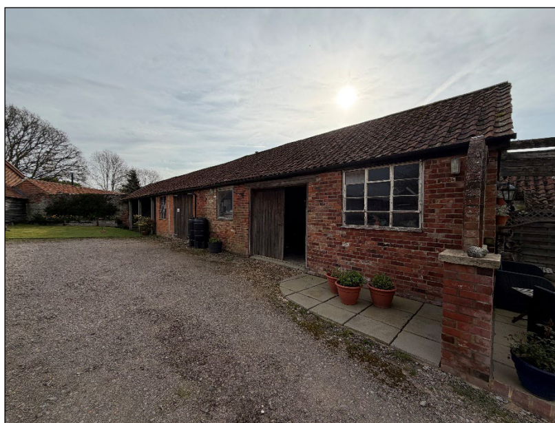
Image 14: Outbuilding viewed from southwest
