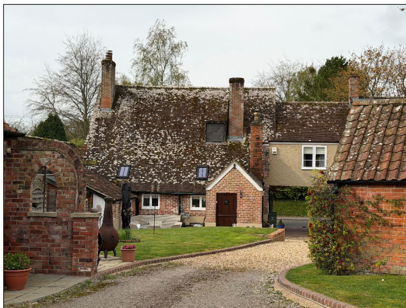
Image 18: No. 69 High Street, rear elevation
