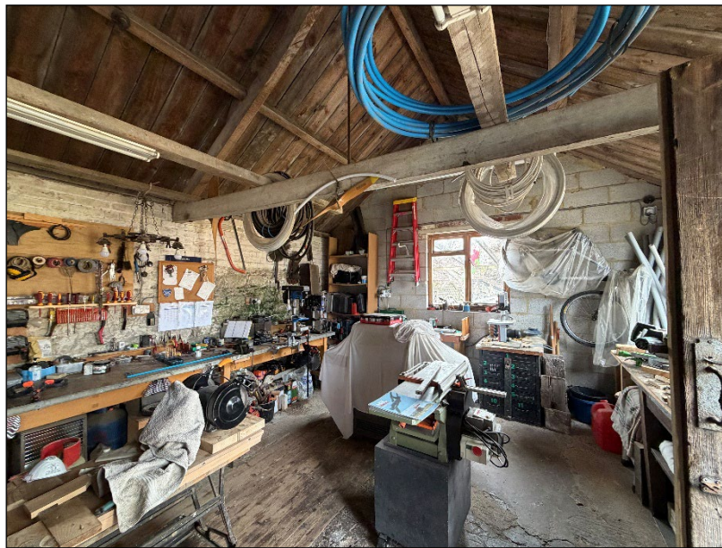
Image 16: Internal view showing replacement roof structure
