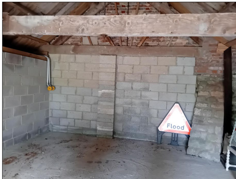
Image 13: Modern infill to rear garage wall
