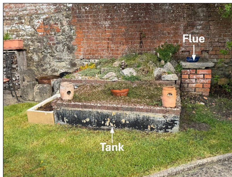
Image 8: Remains of rendering copper system
