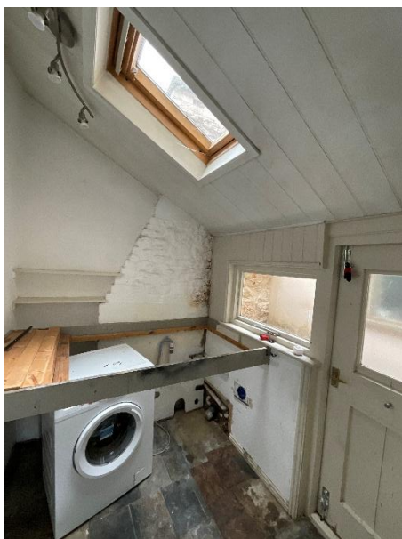
Figure 7 - Existing utility area
