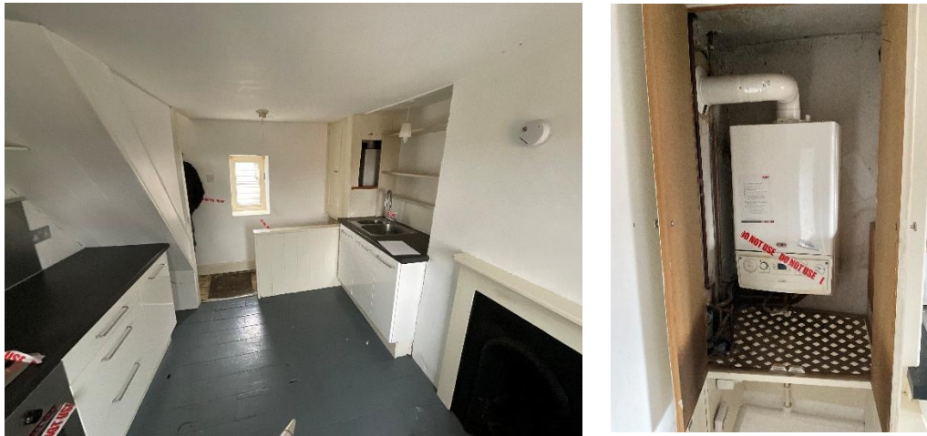
Figure 11 - FF modern kitchen and gas boiler
