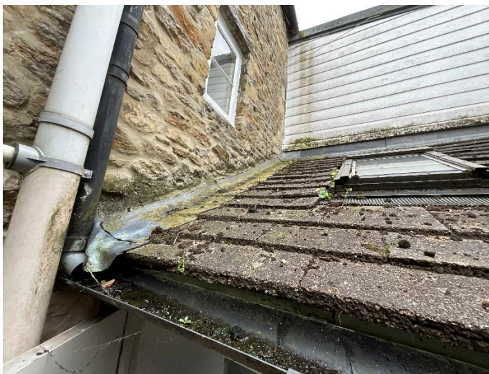
Figure 6 - Existing roof at the rear
