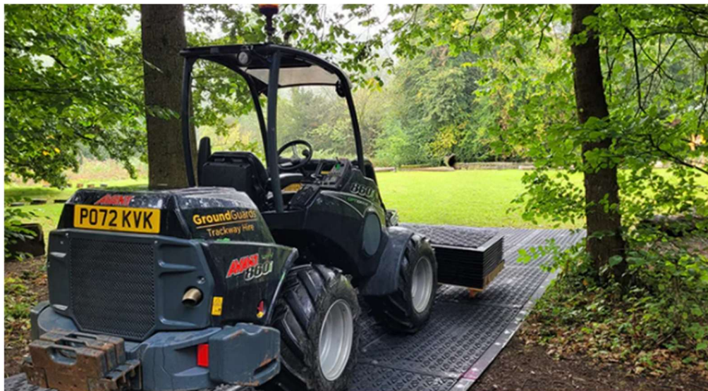
Figure 3: Example of proprietary, inter-linked ground protection boards used as tree root protection.
