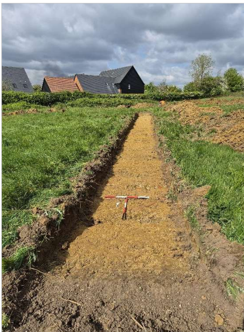
Plate 3: Trench 3 view north. 2 x 0.8m scales.
