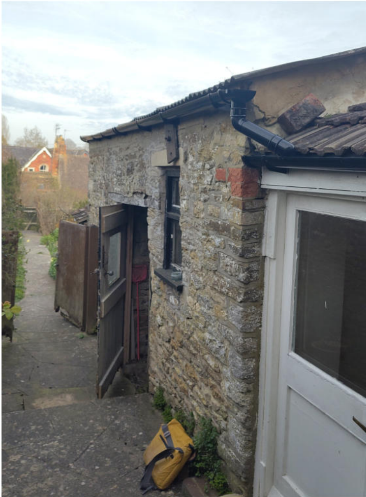
View of the outbuilding. The existing kitchen door can be seen to the right.
