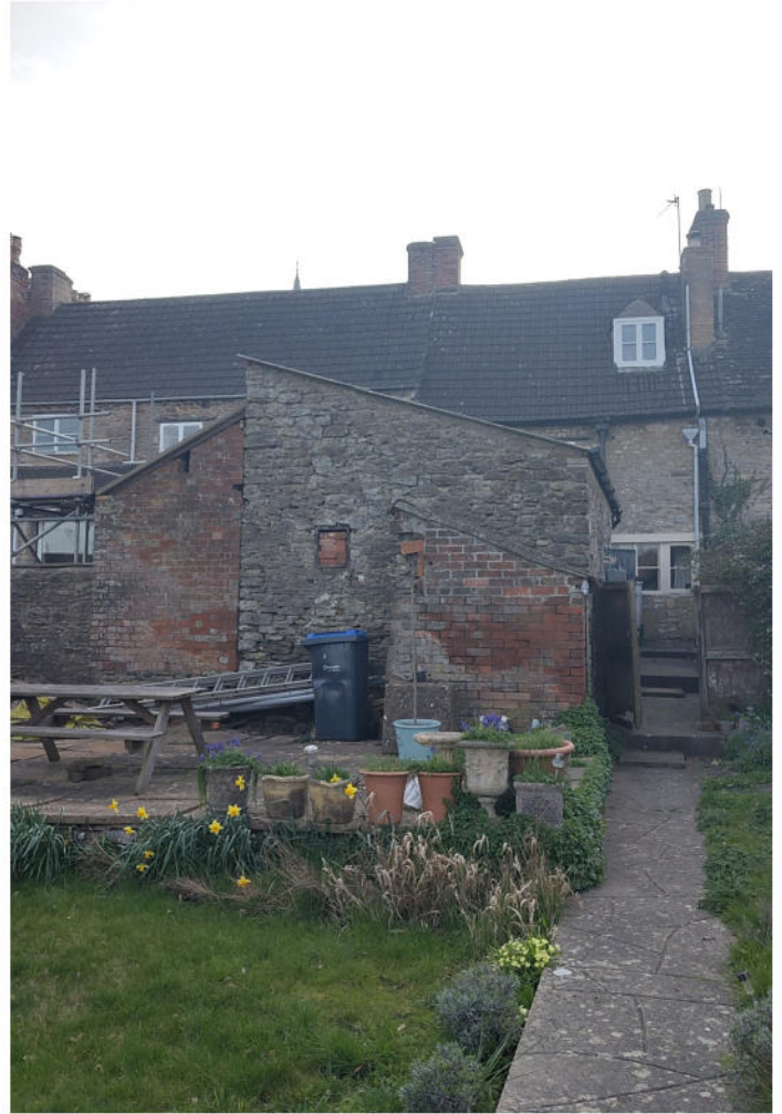
View to the rear showing the existing outbuilding and the neighbouring brick structure to the left. The side access can be seen the right, with dormer window above.
