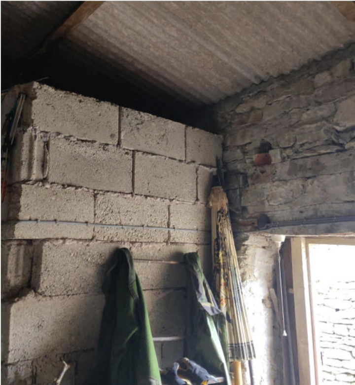
Internal view of the outbuilding showing corrugated roof and modern blockwork
