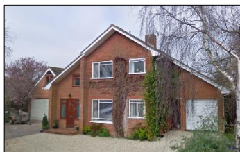
'Catslide' extension to main roof
