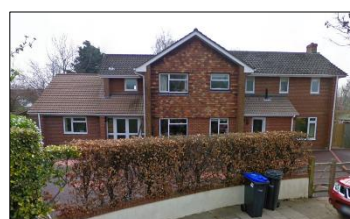
Full height two storey extension
