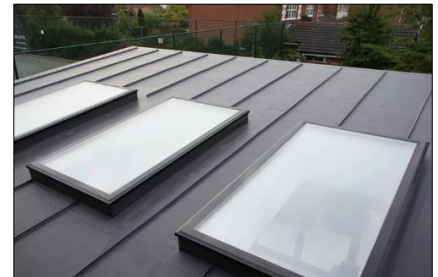
ROOF LIGHTS (in flat roof)
