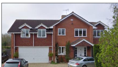
Two story side extension with dormers
