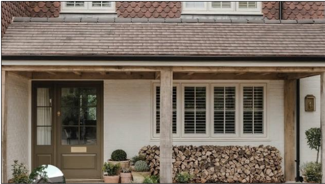
Front canopy and painted brick (Off White)
