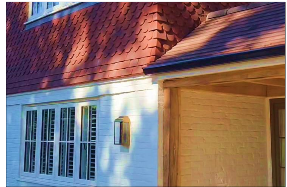
Tile hanging over painted brickwork
