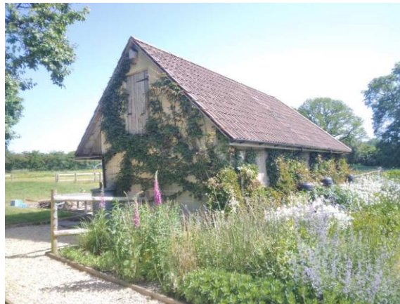
Building B1 - South-western elevation
