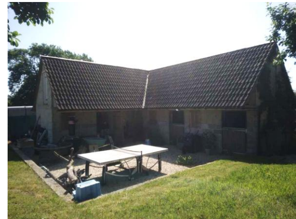
Building B1 - Northern and western elevations
